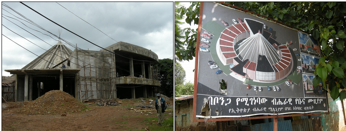
Figure 8. 4 National Coffee Museum Under Construction
