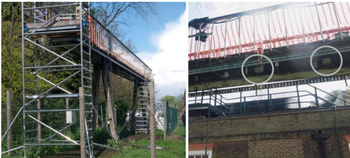
Figure 6.37 Back view of the NPL Footbridge (left) and front view of mid-section of the footbridge (right) with tilt-meters (circled).
