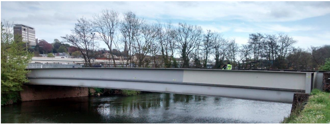
Figure 3.4 North face of the River Exe Bridge.
