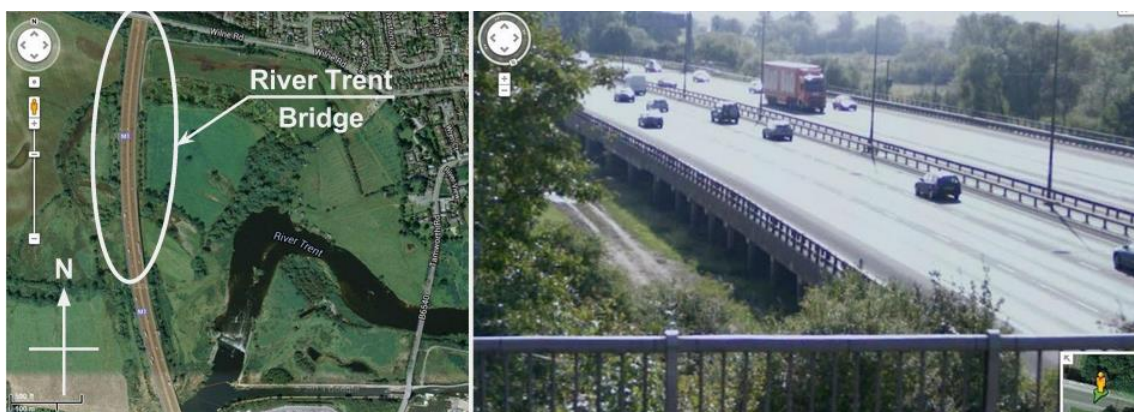
Figure 6.60 Aerial view of the River Trent bridge (left) and a view from an overcrossing (right) [229].
