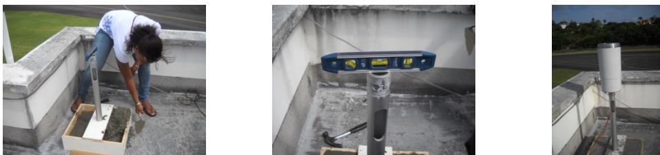
Figure 2-3: Physical installation of the tipping bucket rain gauge
