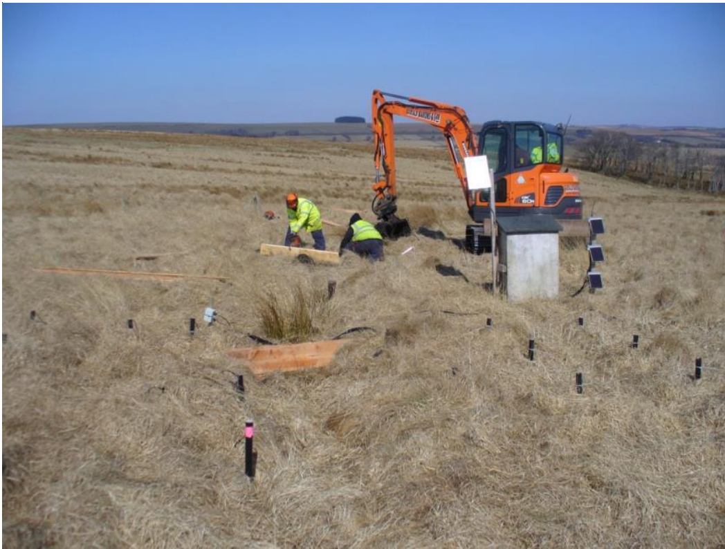
Figure 3.17: Restoration of the S1 monitoring location in the Spooners catchment, March 2013.
