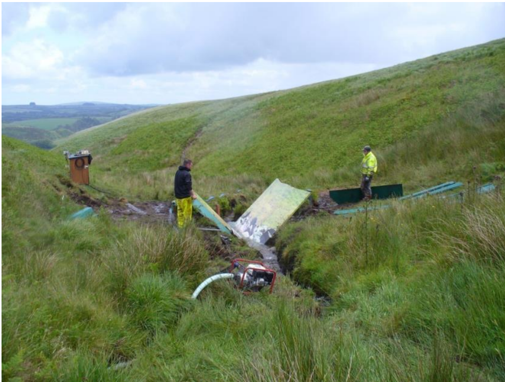
Figure 3.15: Contractors installing the flume structure at the Aclands catchment outlet, Summer 2011.
