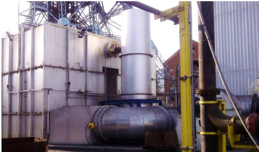
Figure 3.2.4 Hel East VAM abatement RTO design (Courtesy HEL-East)
