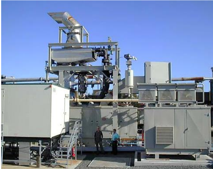
Figure 3.2.2 Appin colliery turbine installation (source, Cummings, 2004)
