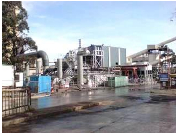
Figure 3.1.4 The West Cliff VAM Project or WestVAMP VOCSIDIZER™, (Courtesy of MEGTEC)
