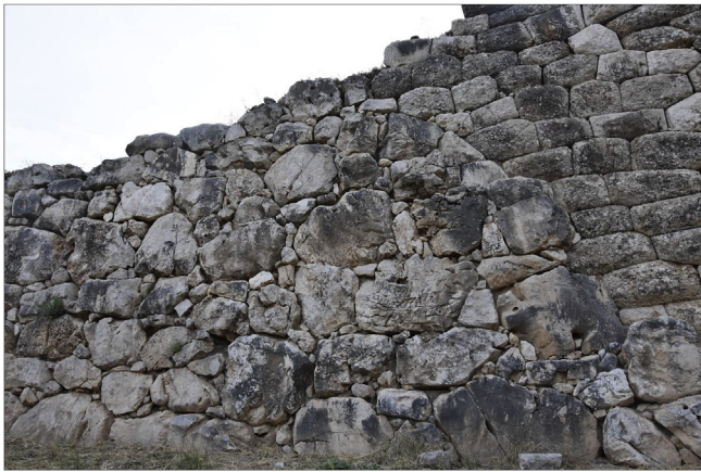
Fig. 13. Mycenae, citadel. A section of cyclopean-style wall with the large boulders and smaller stones in between (left), showing contrast with the well-fitting stones of a later Hellenistic repaired section of the wall (right). (Y. Boswinkel).
