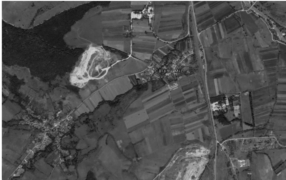
Figure 9 – general view of Călanul Mic – Sâncraii quarry
