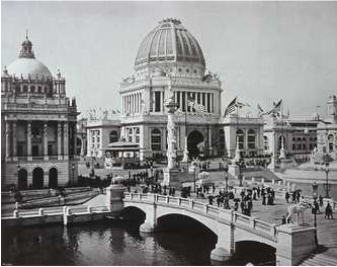
Figure 3: “The Administration Building.”
