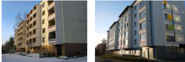
Figure 2. Case study building before and after energy retrofit.
