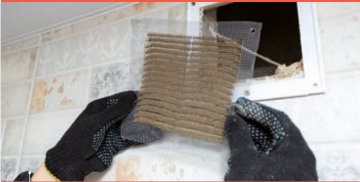
Replacement of a ventilation filter
