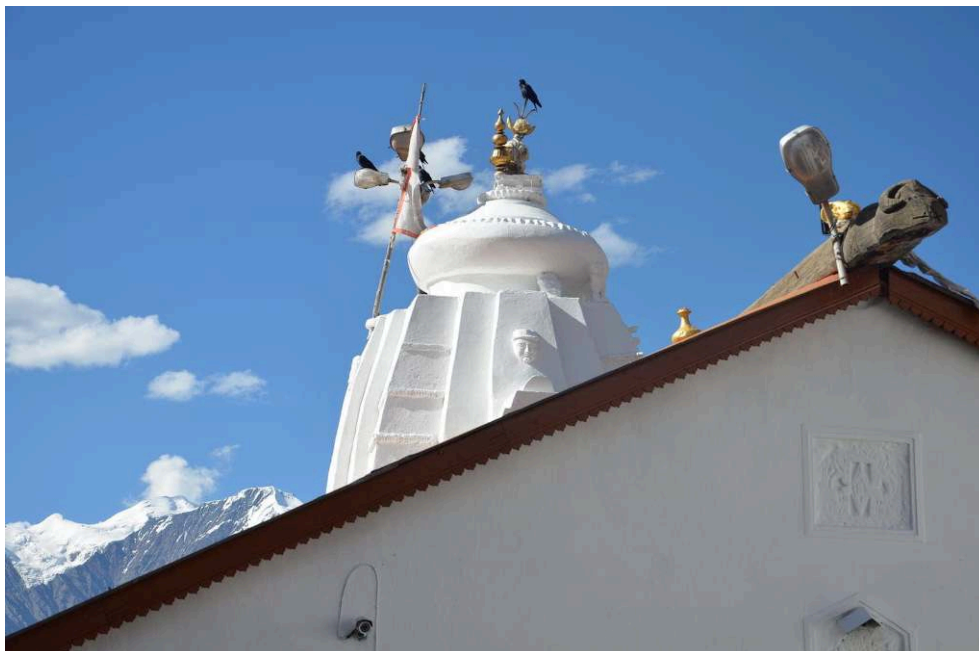
Figure 9. View from the yard
