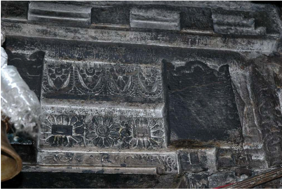
Figure 18. Lintel, right side
