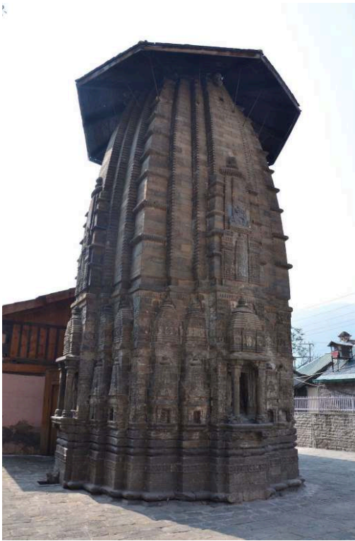
Figure 16. Chamasen Bhagvati temple of Chamba with pranala and high-relief miniature temples extending beyond the kanta
