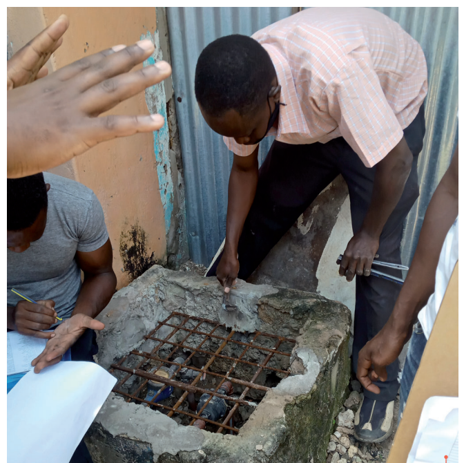
MAWASCO staff oversee commissioning of smart meters - ©UNTAPPED
