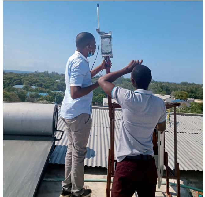
Configuration of smart meter communication antennae - ©UNTAPPED
