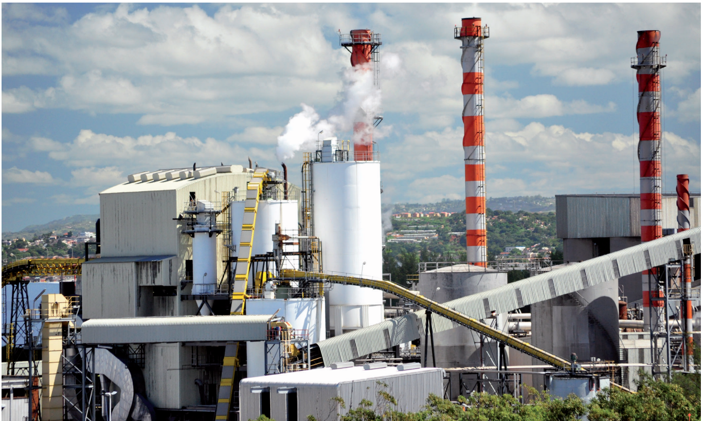
In Durban, wastewater is reused for industrial purposes - ©Veolia
