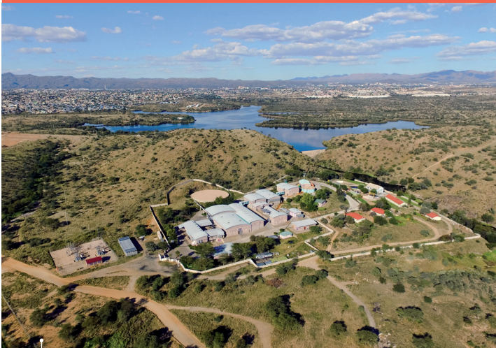
Windhoek wastewater recycling plant - ©Veolia
