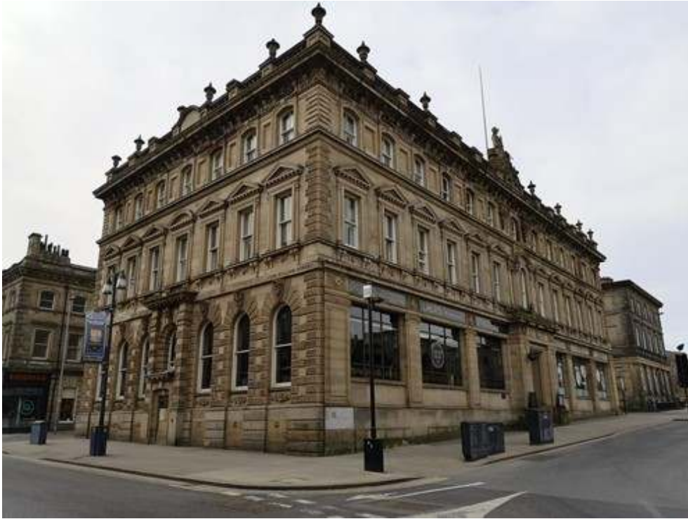
Figure 7. Tite Building, Huddersfield (1851).
