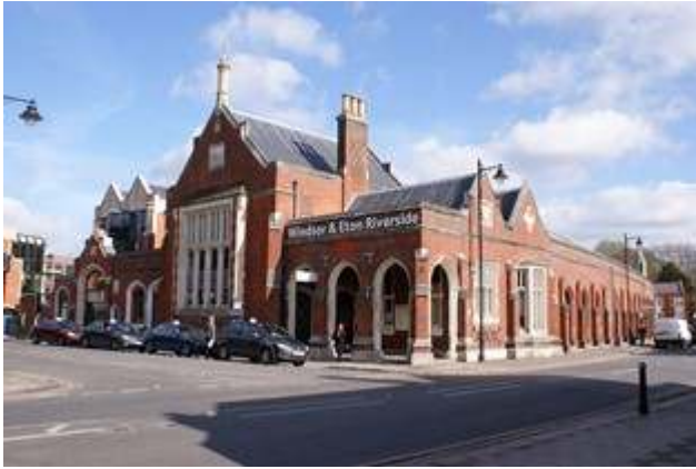
Figure 10. Windsor & Eton Riverside station today.
