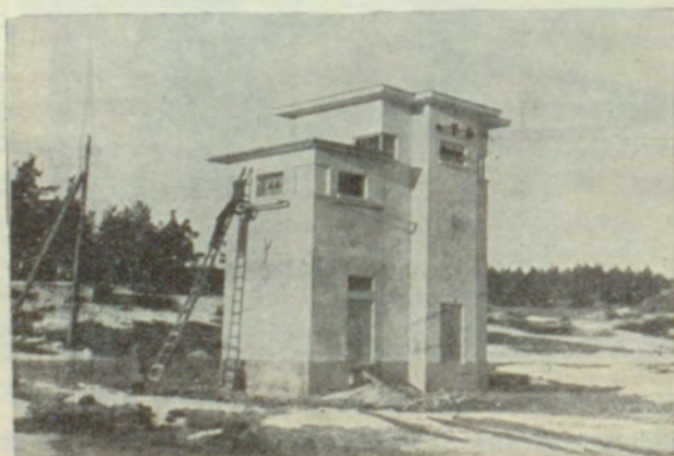
Abb. 19. 20 kV Trafostation.
