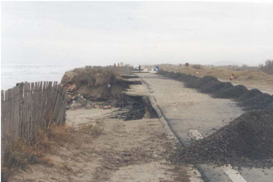
Fig. 4.19 Recurrent erosion impacts on the coastal road
