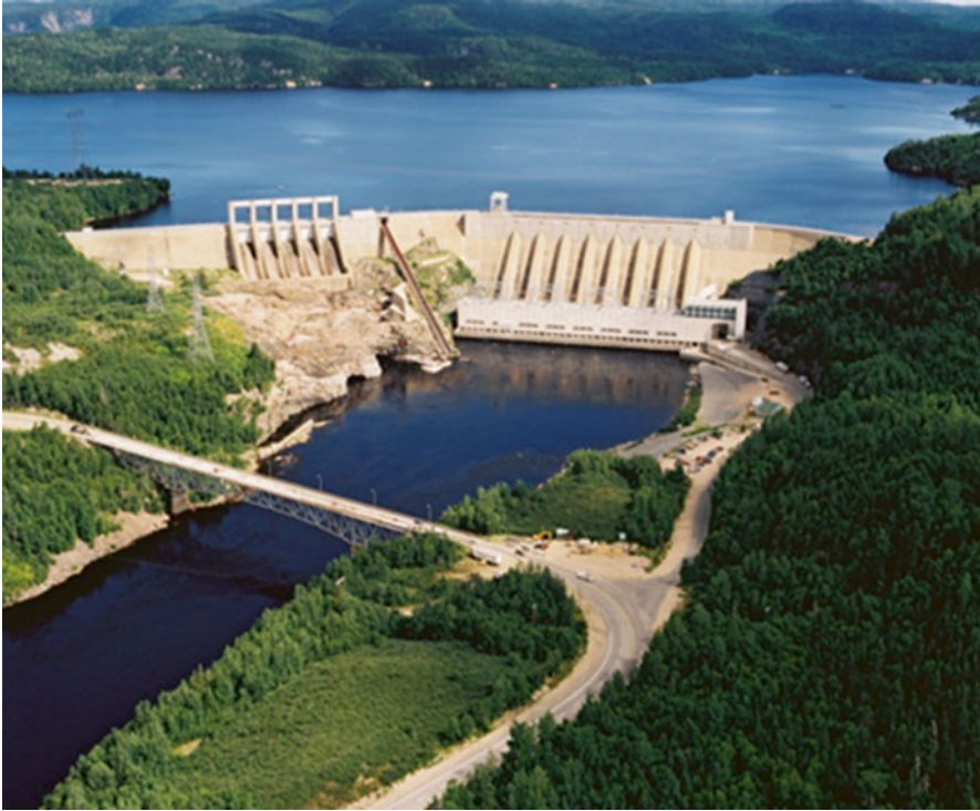
Fig. 4.22 Manic 2 Power House on the Manicouagan River (Source: Hydro-Québec)
