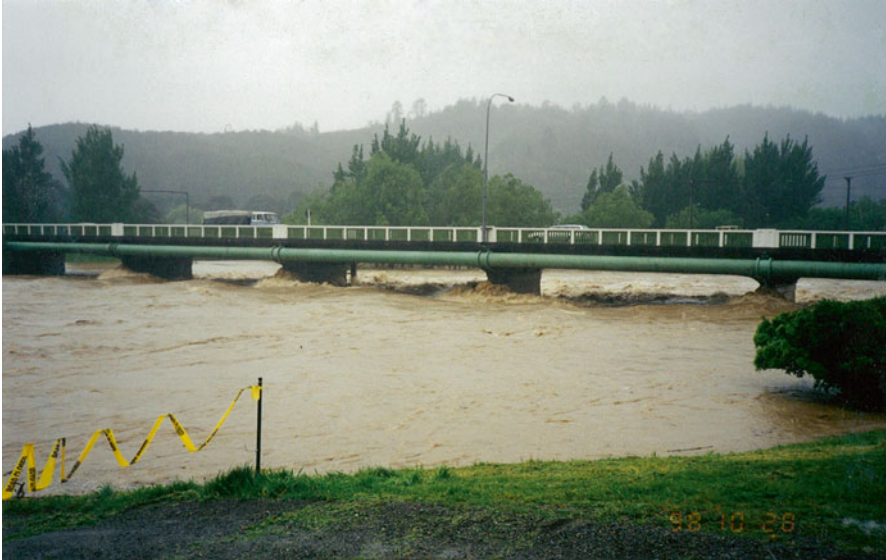
Fig. 4.30 Flooding of the Hutt river
