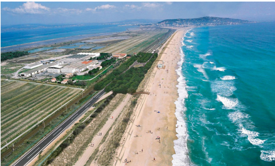
Fig. 4.21 Global overview after completion of the project showing the road moved inland and the restoration of a wider beach and sand dune
