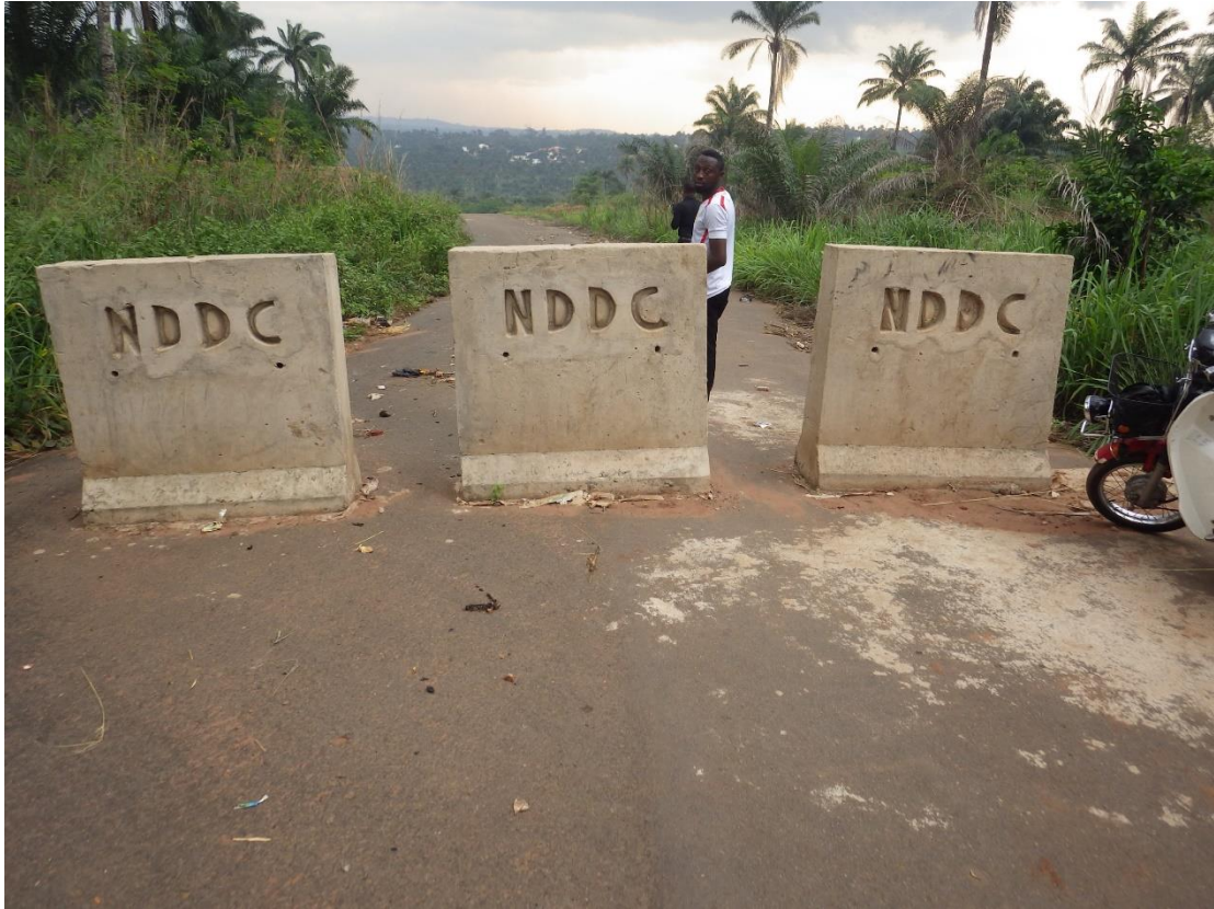
Figure 7.2: Barricades aimed at halting further movement of commuters along the road.
