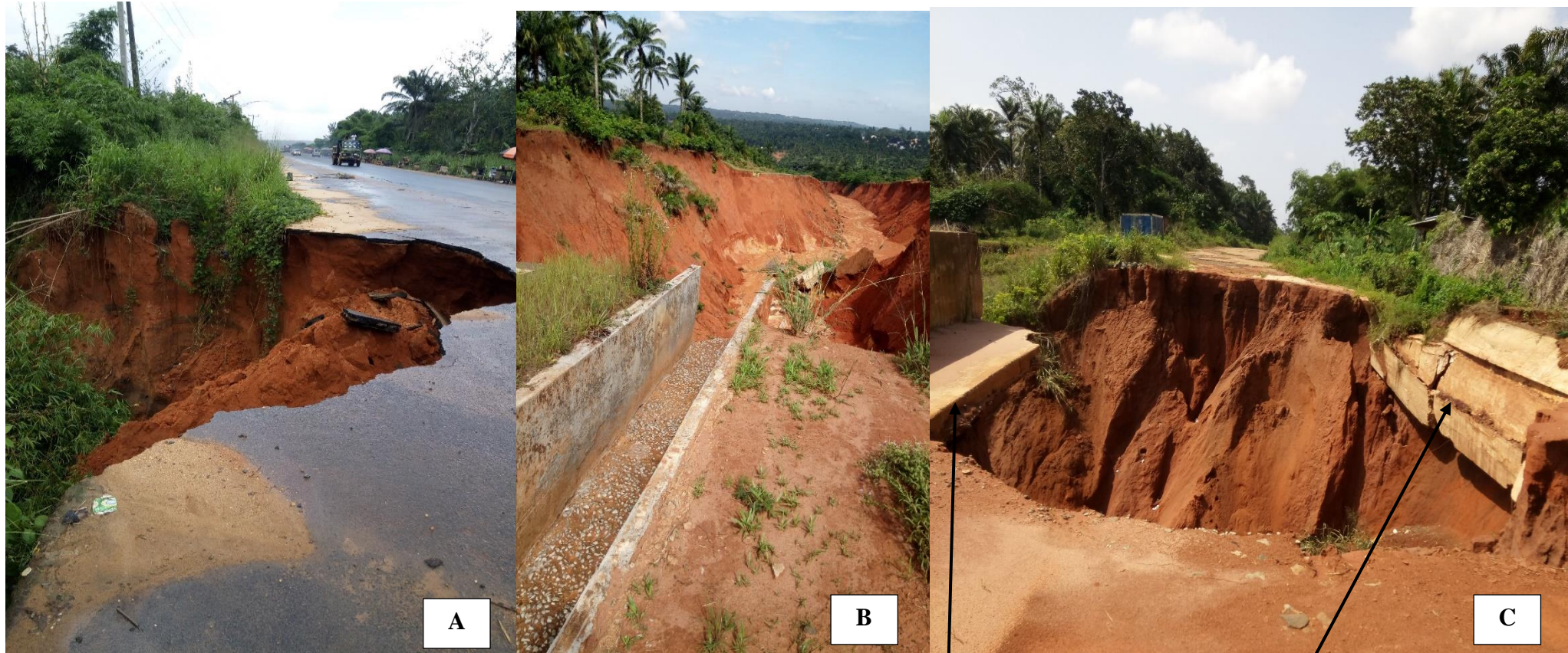
Concrete structure designed for gully rehabilitation
