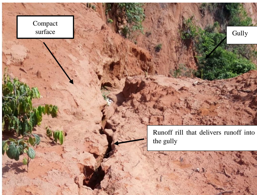
Figure 5.20: Runoff rill formed on compacted surface at the Umueshi abandoned gully rehabilitation site. Rills found close to gullies had depth ranges between 0.4 – 0.7 m, widths varied between 0.25 & 2.2 m while lengths ranged from 10 – 60 m.
