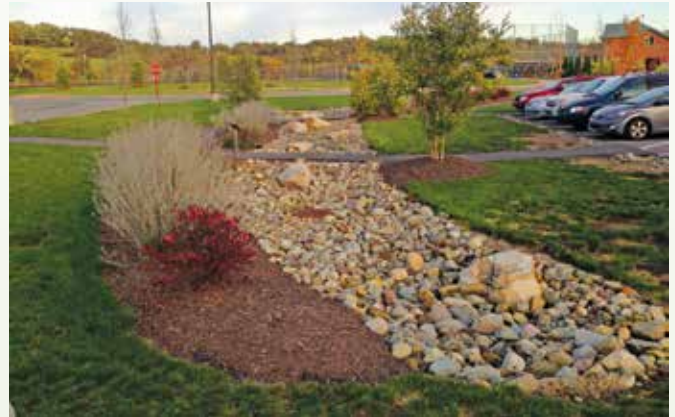
Photo courtesy 3 Rivers Wet Weather
