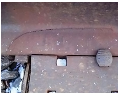
Figure 1. Longitudinal foot flaw (half-moon defect)
