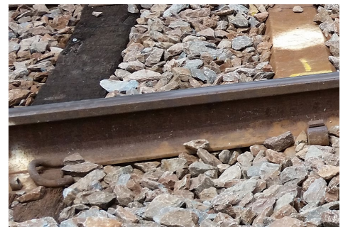
Figure 3. Example of obstructions in the foot region
