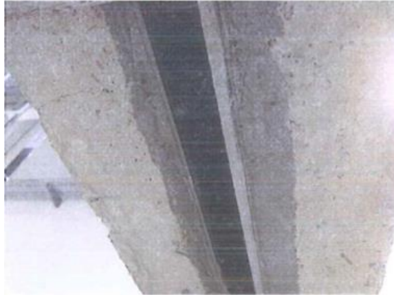
Fig. 4. Type of pasted composite
