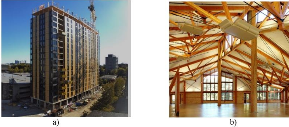
Fig. 1. Wood frame buildings: a) Student residence in Canada; b) Interior of the Hayden Camp dining hall, USA, owned by the Fresh Air Fund's.
