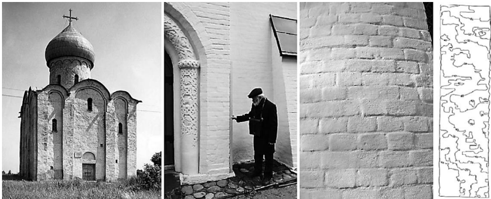
Fig. 10. Relief of the facade of the Church of the Saviour on Neredita after the restoration of 1958; photo Borovaya E.L., Zommer T.V.: relief of the portal of the Church of the Image of Edessa in Abramtsevo; map of the buttress surface relief [4]
