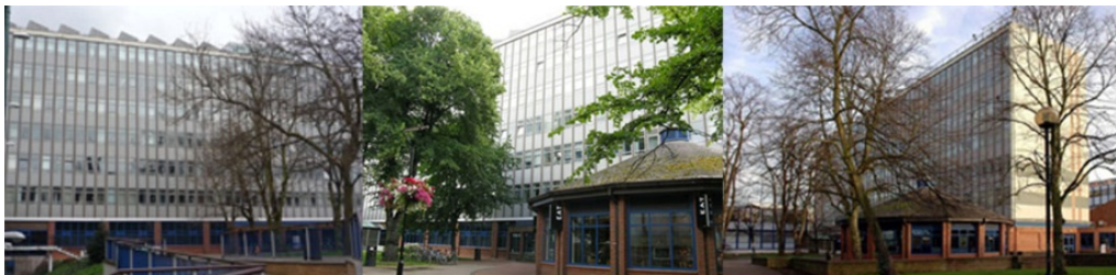
Figure 10 - External view of George Eliot Building
