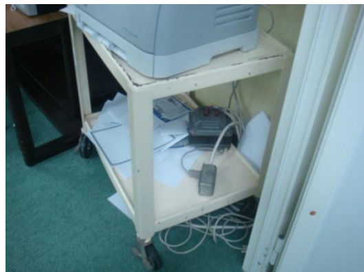
Exposed wiring
