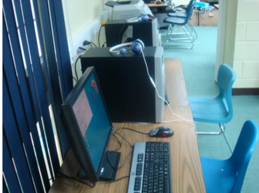
Inappropriate location of terminals
