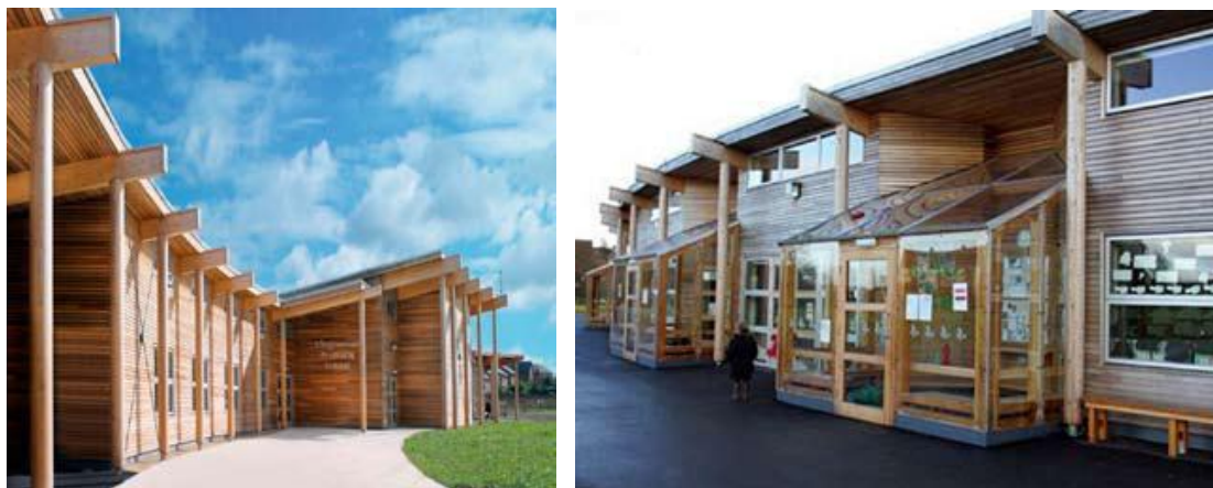
Figure 2.2 : Timber on all the elevations to give a rustic and unified character (Kingsmead Primary school)
