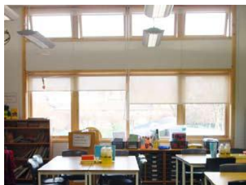
Figure 2.8 - Small windows at the top allowing ventilation Without draught (Rolls crescent Primary school, Manchester, UK)
