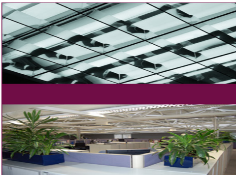
Fig1.18: Cleaning could restore light its design level.
