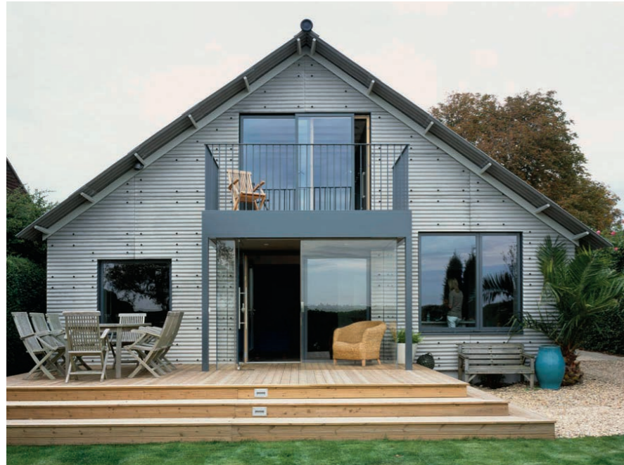
Fig. 28 Front view of Cement House, clad in corrugated cement board for lichen to grow on.
