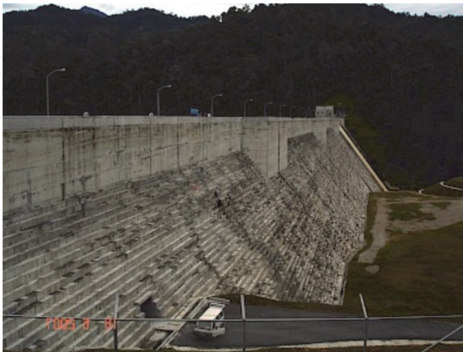
Figure 1. Location of Kinta RCC dam.
