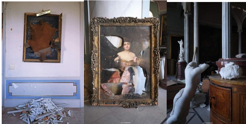
Fig.12: cultural heritage damaged on Sursok museum. Source: Facebook page of Sursok museum.
