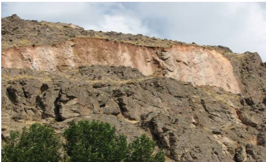
Figure 1.1 Landslide in Atashgah-e- Karaj 2008
