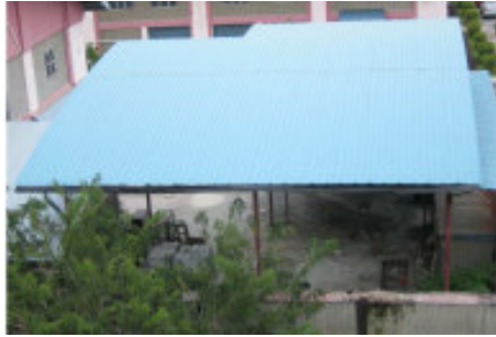
Figure 3: The rainwater catchment comprises of a 100 m 2 roof.
