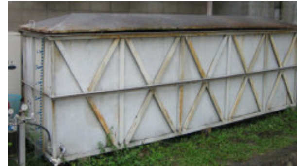
Figure 1: General view of the storage tank.
