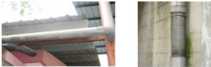
Figure 5: Rain pipe connections and example of a flexible hose.
