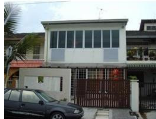
Figure 2: Front facade of the case study building.
