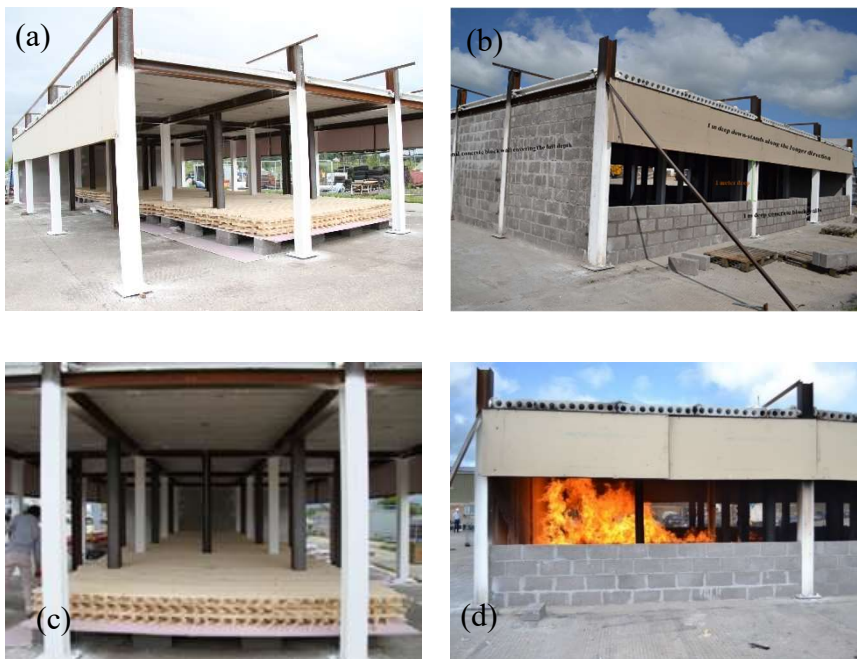
Figure 2 - Photographs of the experimental campaign carried out by Ulster University in the frame of TRAFIR project: (a) compartment for test n°1 ; (b) compartment for test n°2 ; (c) continuous fire load made of wood sticks for test n°1 and test n°2 ; (d) fire at the beginning of test n°2
