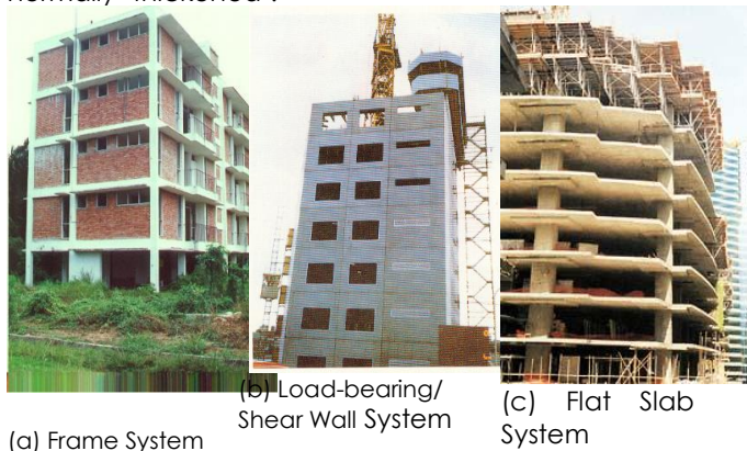
Figure 1 Building structural systems
