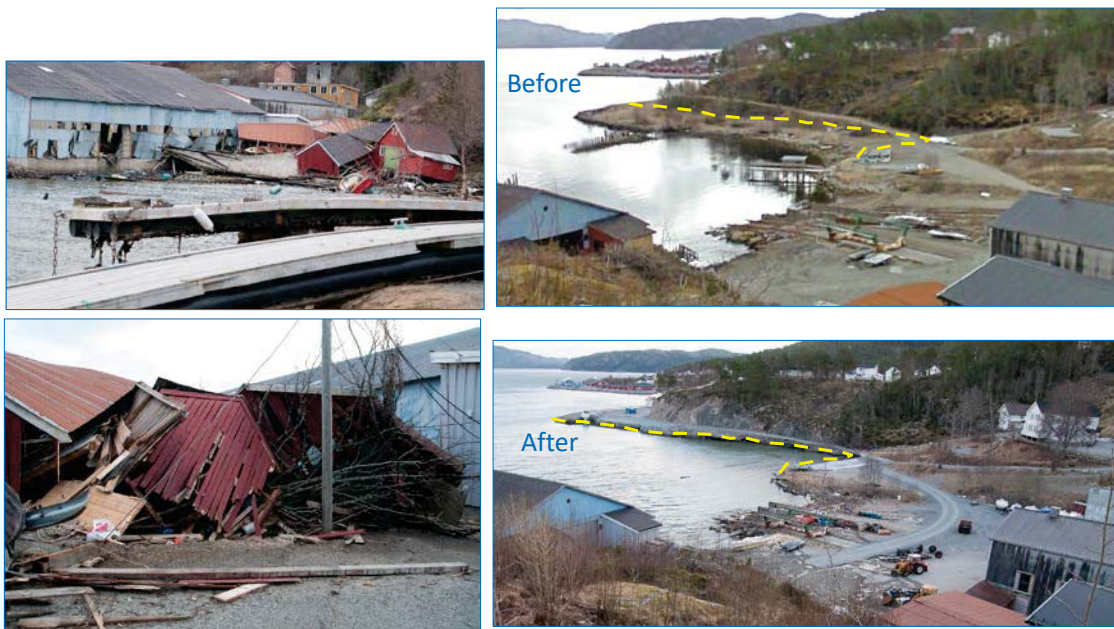
Figure 1 Photos showing damage caused by the Statland landslide. The right hand side photos compare the situation before and after the landslide with yellow dashed line showing the shoreline after the slide.
