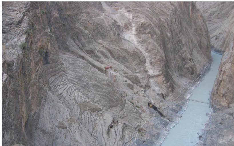
Fig. 1. Bakhtiary dam location [10].
