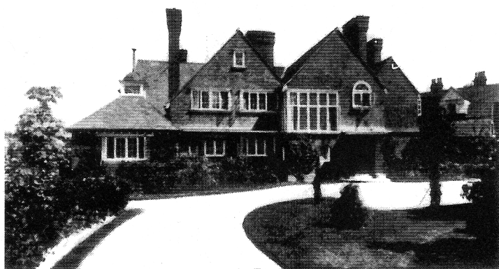
42 The Gables, Esher, Surrey. By Seth Smith. View from forecourt
