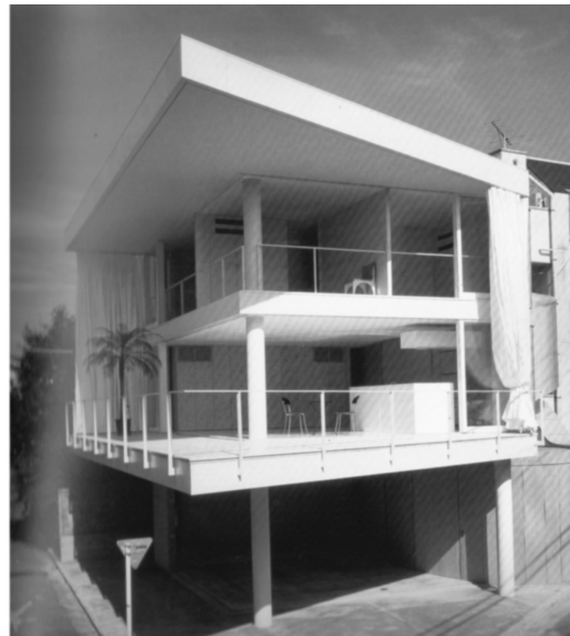
Fig. 4. Curtain Wall House with curtains open, Tokyo 1995, in Terence Riley, The Un-Private House (New York: The Museum of Modern Art, N.Y., 1999) 73.
