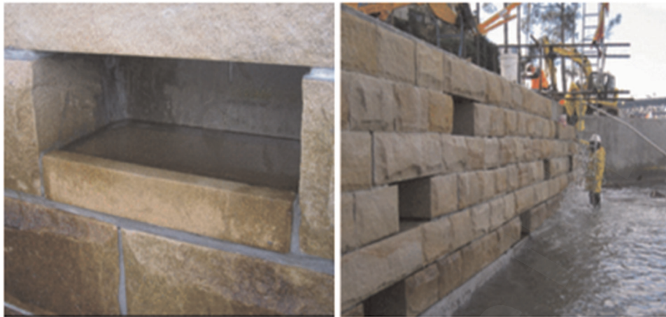
Fig. 7 Built-in rock pools in Sydney Harbour walls. Source: [35]
