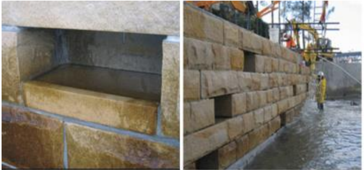
Figure 30 Built in rock pools in Sydney Harbour walls. Source: [212]
