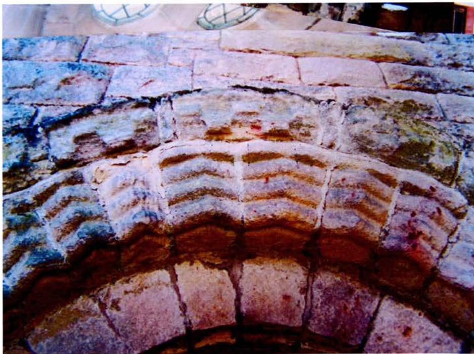
18) Bridekirk (St Bridget) : east doorway of south transept
