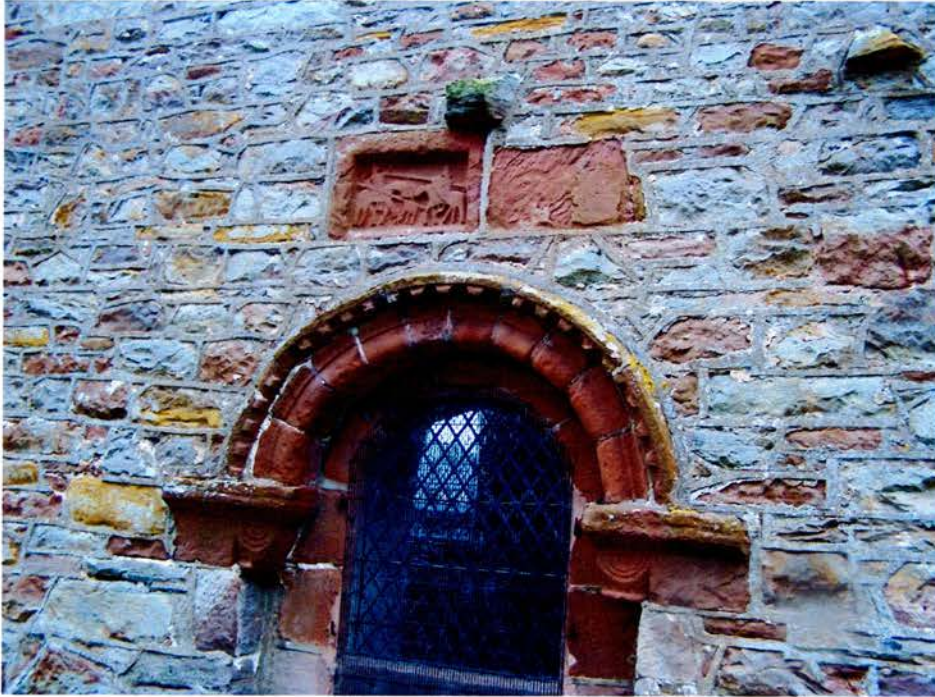
3) Bolton (All Saints) : two reliefs in north wall
