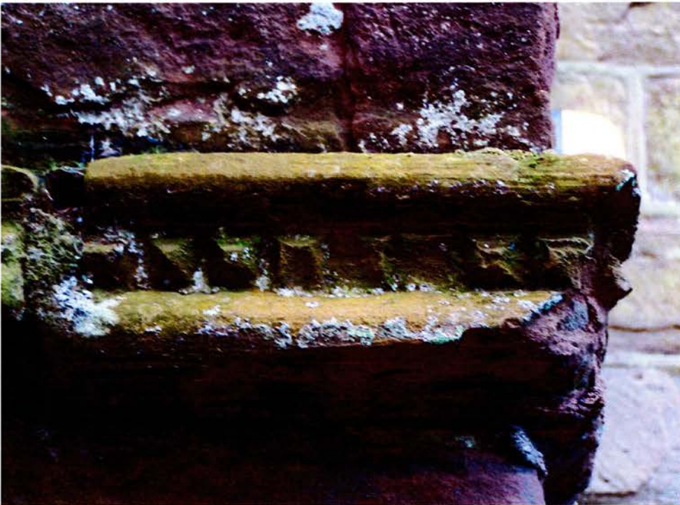
120) St Bees (St Mary and St Bega) : string-course fragment, east side of north transept
