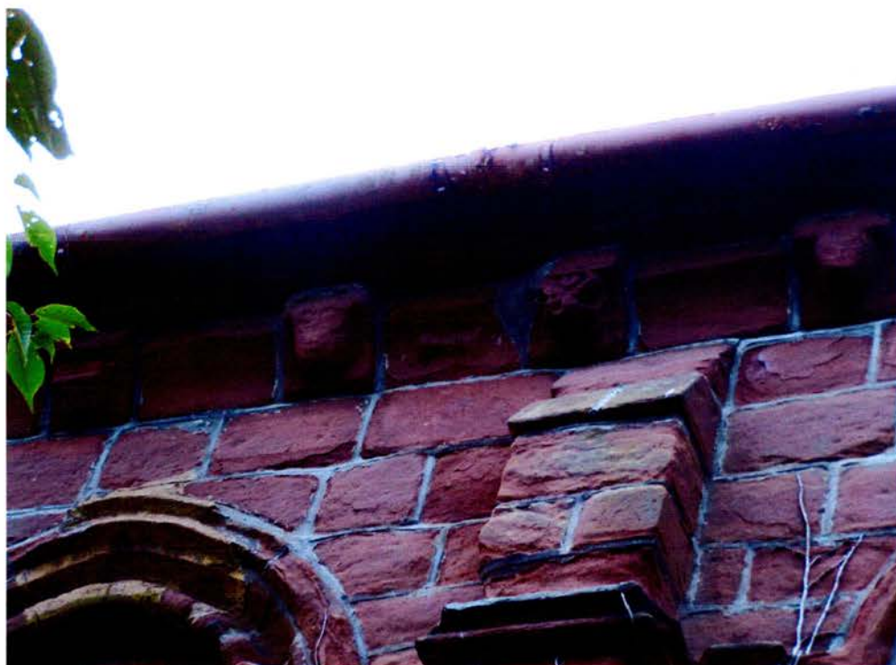
118) St Bees (St Mary and St Bega) : corbel-table, north side of nave, detail
