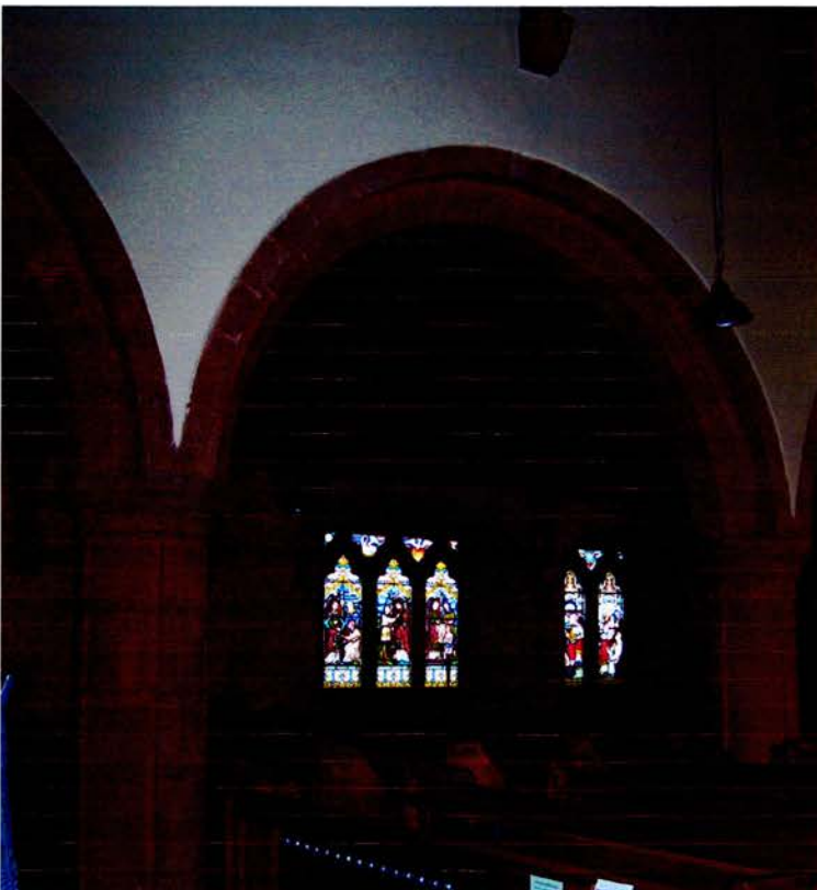
41) Bromfield (St Mungo) : pier in nave
