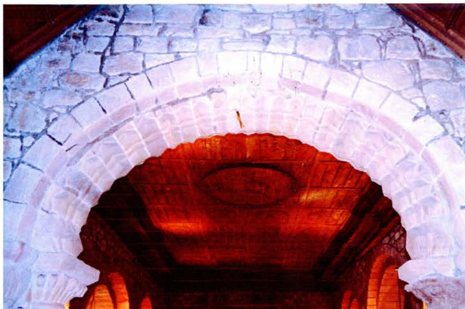
134) Torpenhow (St Michael) : chancel arch from east
