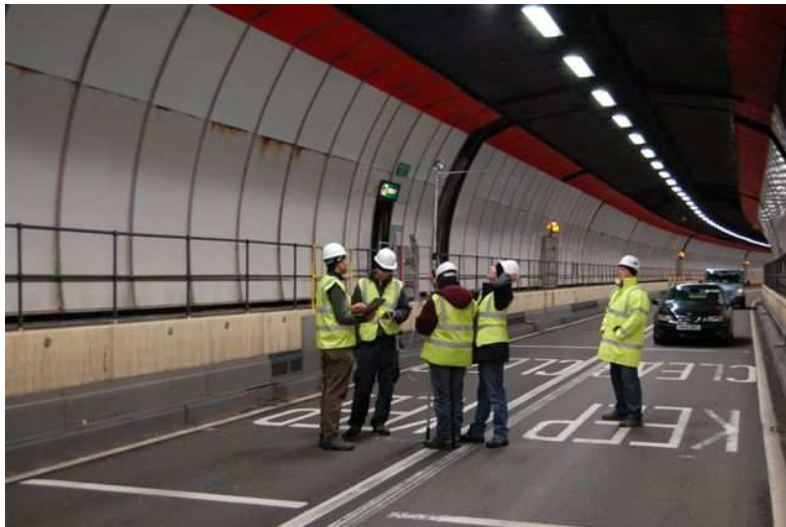
Figure 48: West Dartford Tunnel; Picture taken approximately 500 m from the Kent portal facing south (refer to Figure 46).
