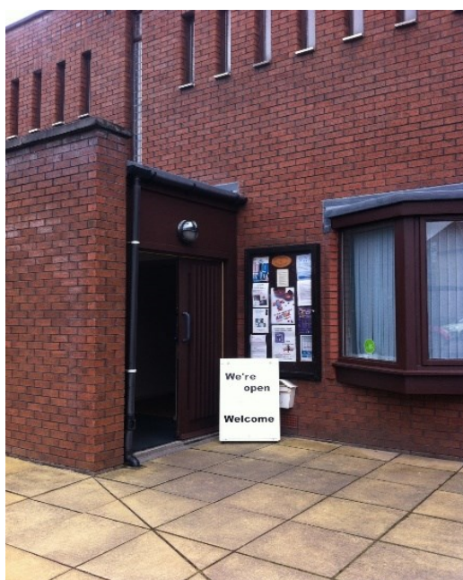
Figure 4.1 Entrance to Saughtonhall Church
