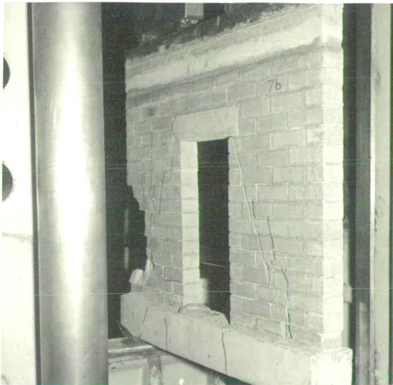
PLATE 7.2 CRACK PATTERN IN WALL 7b AT ULTIMATE LOAD
