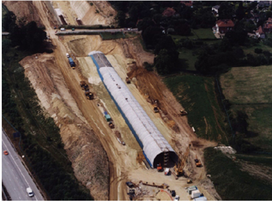
Figure 8.10 - Construction of the Eyehorn tunnel
