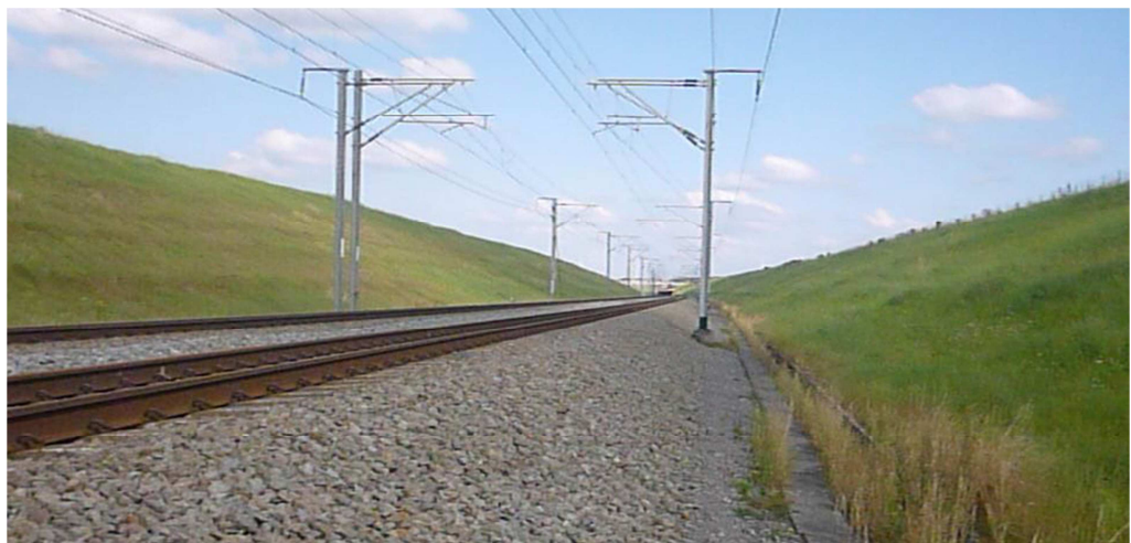
Figure 8.6 - Belgian cutting test site
