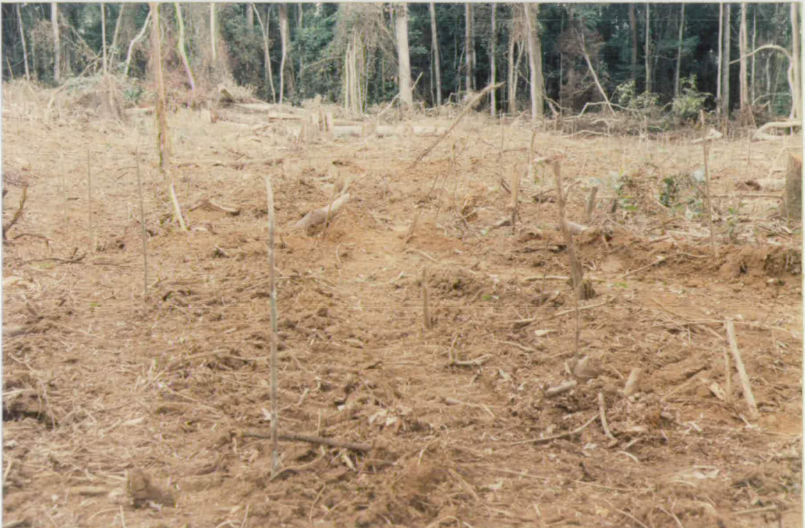
Plate 4: Land situation after clearing using the Complete Clearance method. Soils are completely exposed to maximum climatic and environmental effects. Note the compaction resulting from the bulldozer tread lines.
