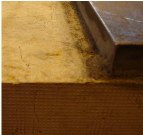
Figure 5.33: Discrete transverse cracking at column location (Slab A, Test A.1 shown).
