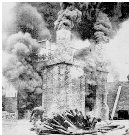
Fig. 1 Early ‘furnace’ test circa 1902 (Stewart and Woolson, 1902)
