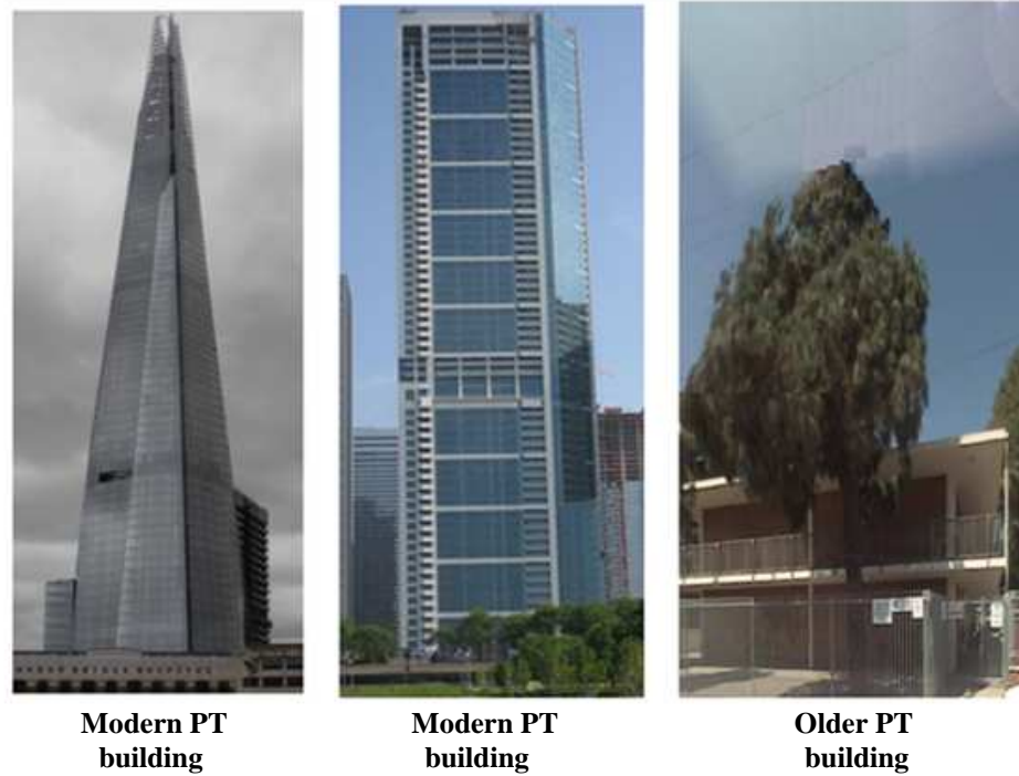
Figure 1.1: Modern versus older PT concrete buildings.
