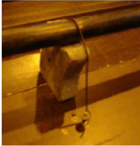
Figure 5.17: Unbonded tendon on a concrete chair tied down to form work.
