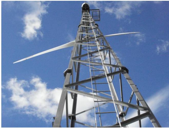
Figure 7.5: Gaia wind turbine with lattice tower configuration
