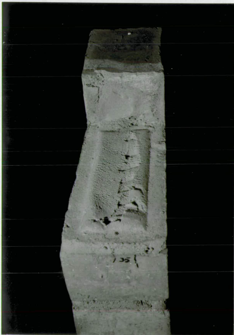
Figure 3.10 - Central Gap in the Mortar Joint (Wall No. 6)
