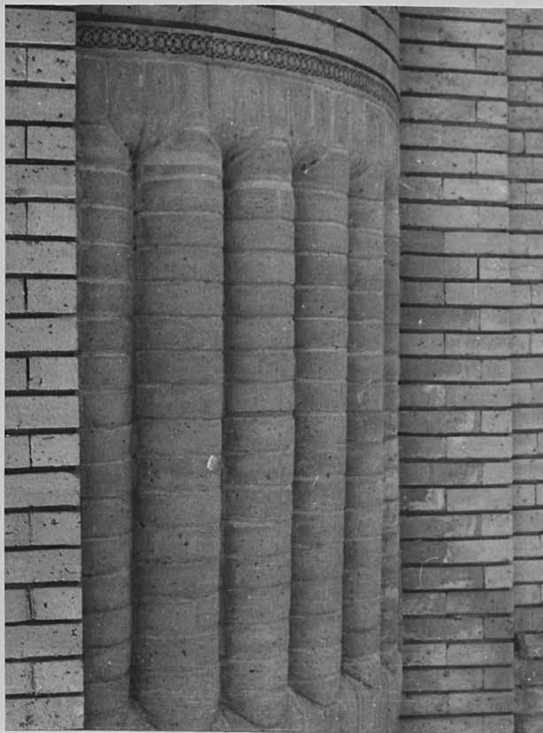
104. Baghdad. Al-Madrasa al-Mirjāniya: exterior. Main entrance: engaged columns on the base of a pier on left-hand side.
