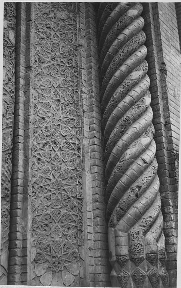
101. Baghdad. Al-Madrasa al-Mirjāniya: exterior. Main entrance: detail of cable moulding and terra-cotta on right-hand side.
