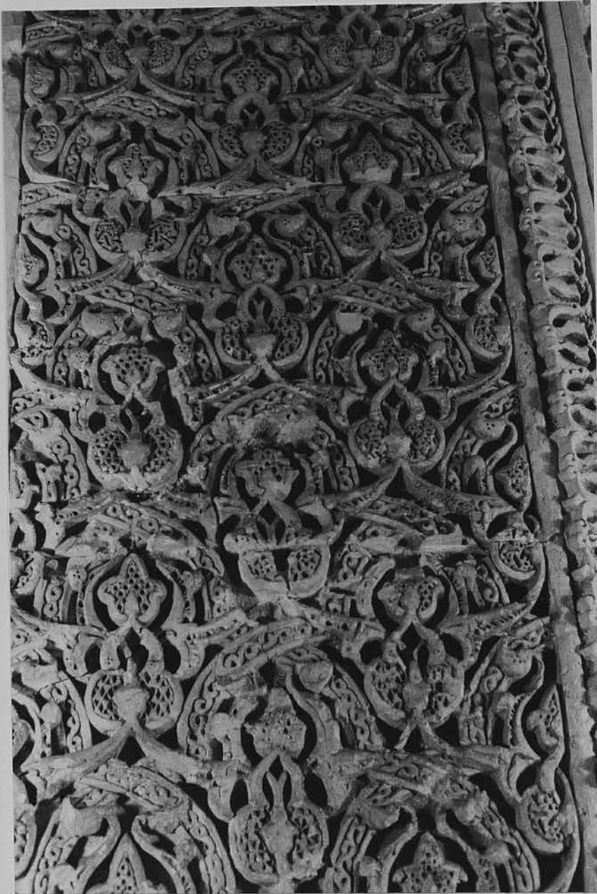
186. Mosul. Al-Nūrī Mosque: interior. Stucco window-frame inside the muṣallā : detail of the left-hand panel.
