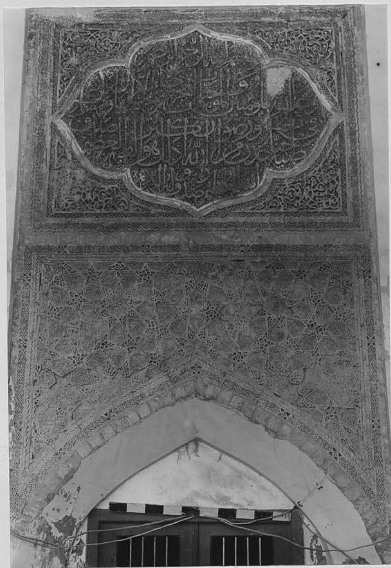
123. Baghdad. Al-Madrassa al-Mirjāniya: musallā façade. Doorway and brick ornament of staircase 6.
