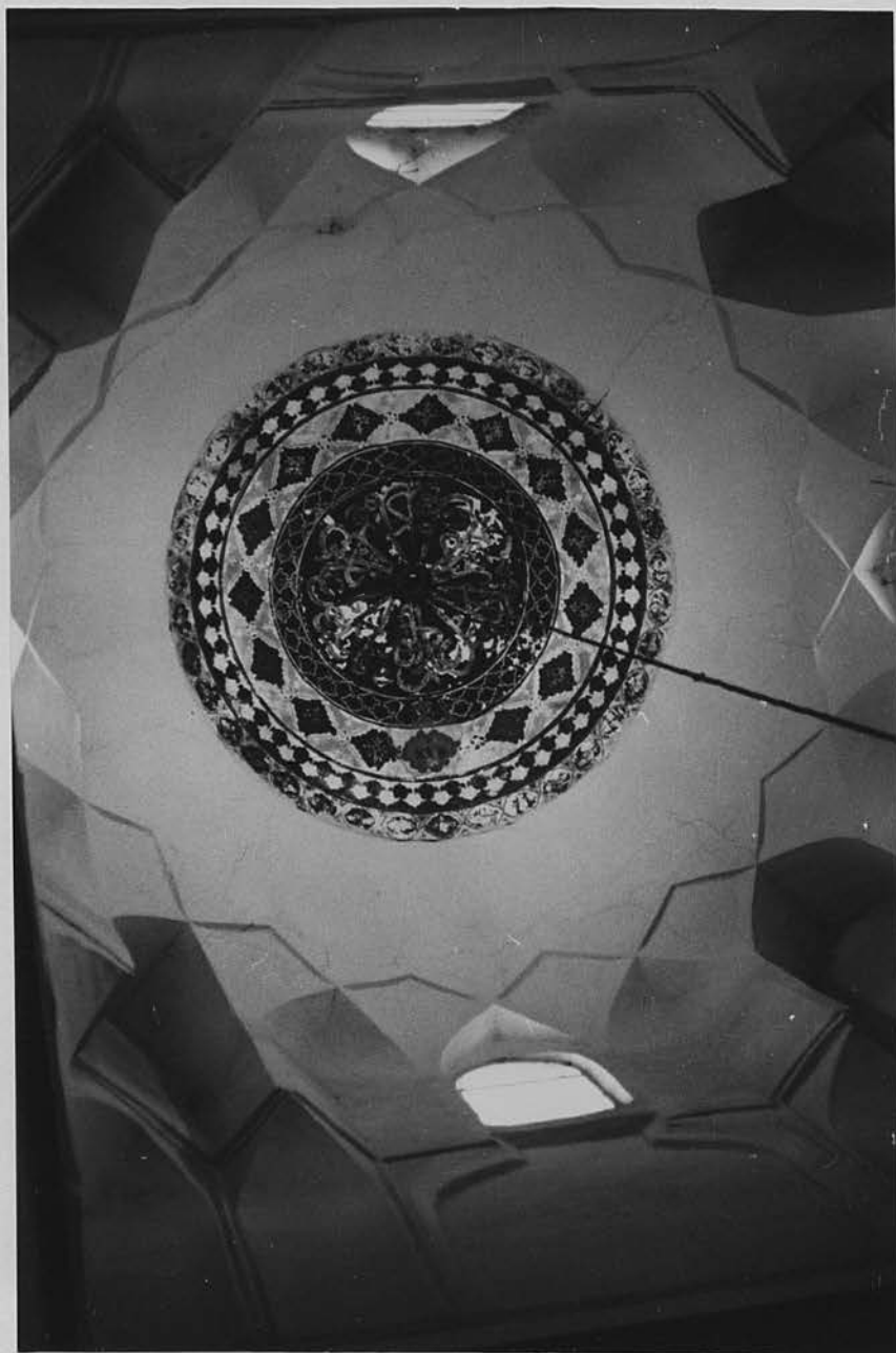
91. Baghdad. The mausoleum of Shaikh 'Umar al-Suhrawardi: interior, showing inner shell of dome and zone of muqarnasat .
