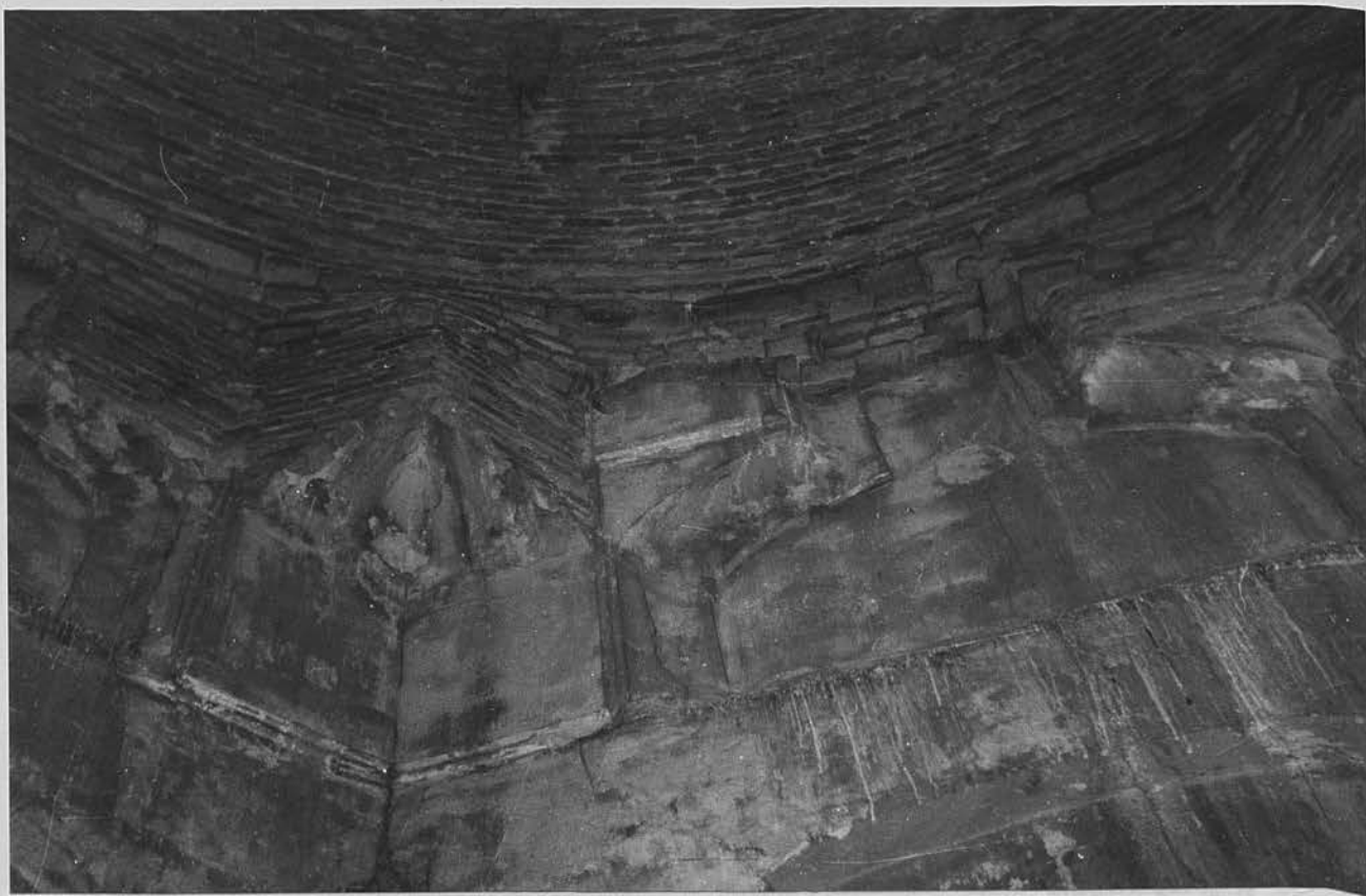
56b. Al-Jadīda (30 km. N.E. of Baghdad): mausoleum of Muḥammad al-Sakrān. Interior: zone of transition, detail of squinch on N.W. side.
