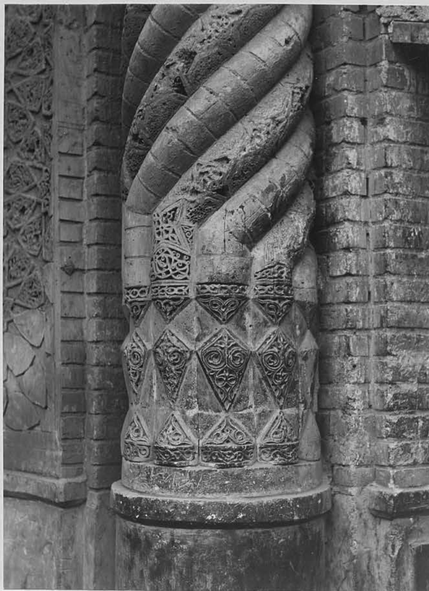
102. Baghdad. Al-Madrassa al-Mirjāniya: exterior. Main entrance: detail of lower part of cable moulding, right-hand side.
