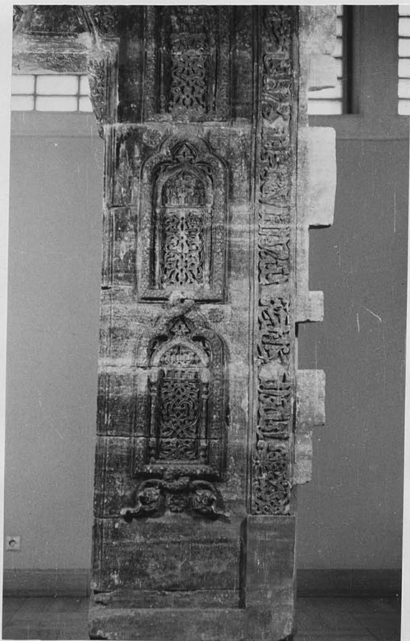
171a. Mosul. Mausoleum of Imām Bāhir: doorway. Detail of the right-hand side.
