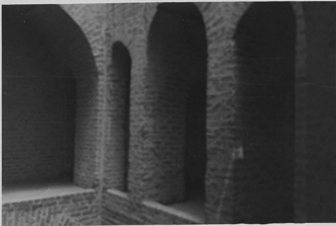
42a. Baghdad. Al-Madrassa al-Mustansiriya: interior of the kitchen; first floor showing triple-arched façade at the N.E. side.
