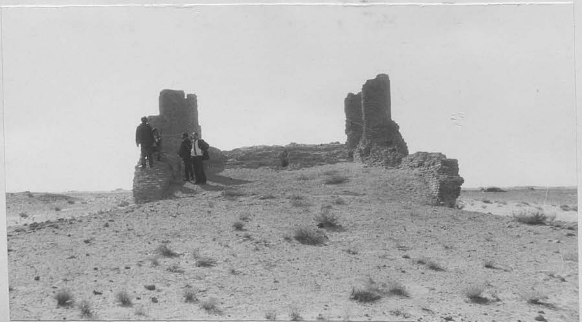
155b. Kūfa. The bridge of Kirī Si'da: roadway, east side.
