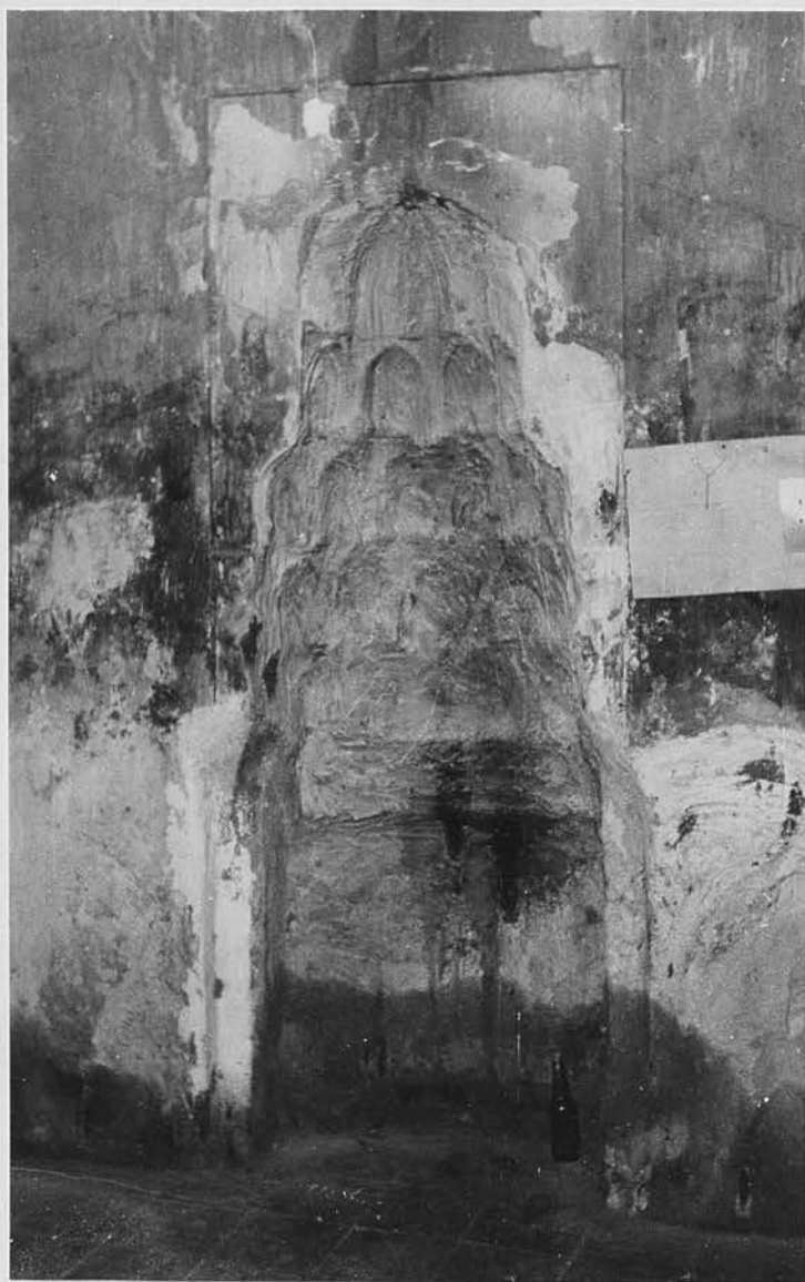
58. Al-Jadīda (30 km. N.E. of Baghdad): mausoleum of Muhammad al-Sakrān. Interior: the mihrāb .
