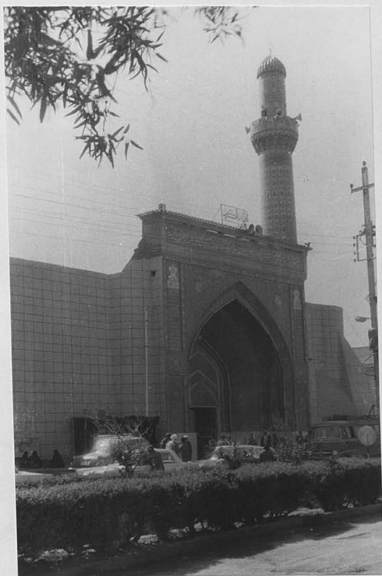
146a. Kūfa. The Great Mosque: the entrance after restoration.
