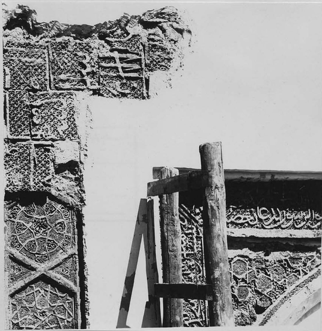
107. Baghdad. Al-Madrasa al-Mirjāniya: interior. Main entrance: detail of terra-cotta.
