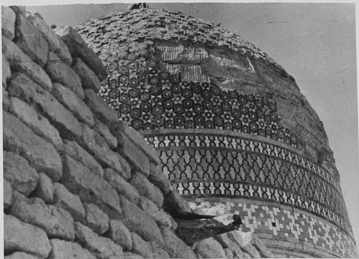
157a. Basra. Jāmi' al-Kawwāz: exterior of dome showing detail of the tile decoration.
