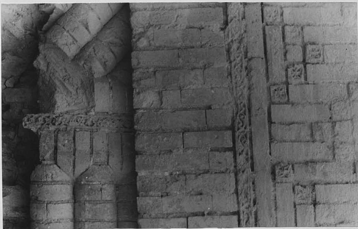
35a. Baghdad. Al-Madrasa al-Sharābiya (the so-called "Abbasid Palace"): brick ornament on western façade; detail of the lower part.
