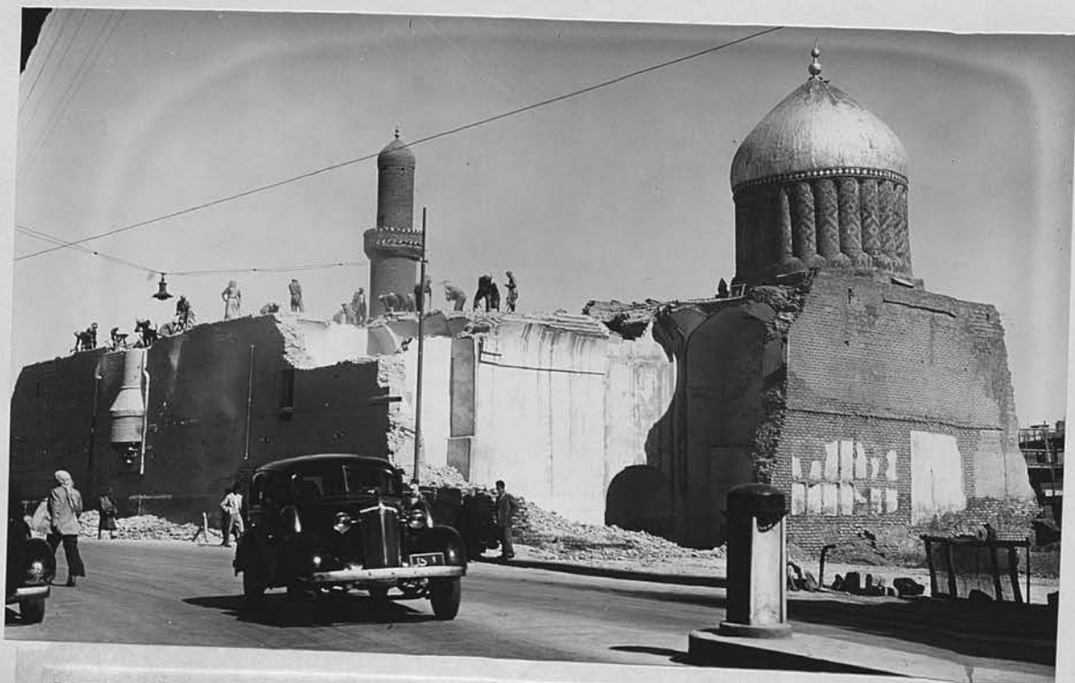
133b. Baghdad. Al-Madrasa al-Mirjāniya: the demolition of the muṣallā . South-west side.
