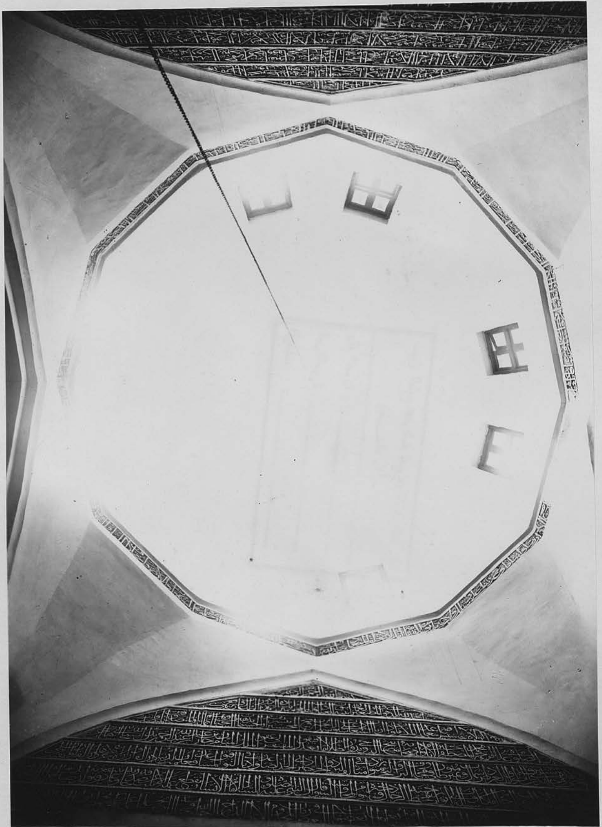
113. Baghdad. Al-Madrassa al-Mirjāniya: interior of the muṣallā , showing inner shell, and zone of transition of middle dome.
