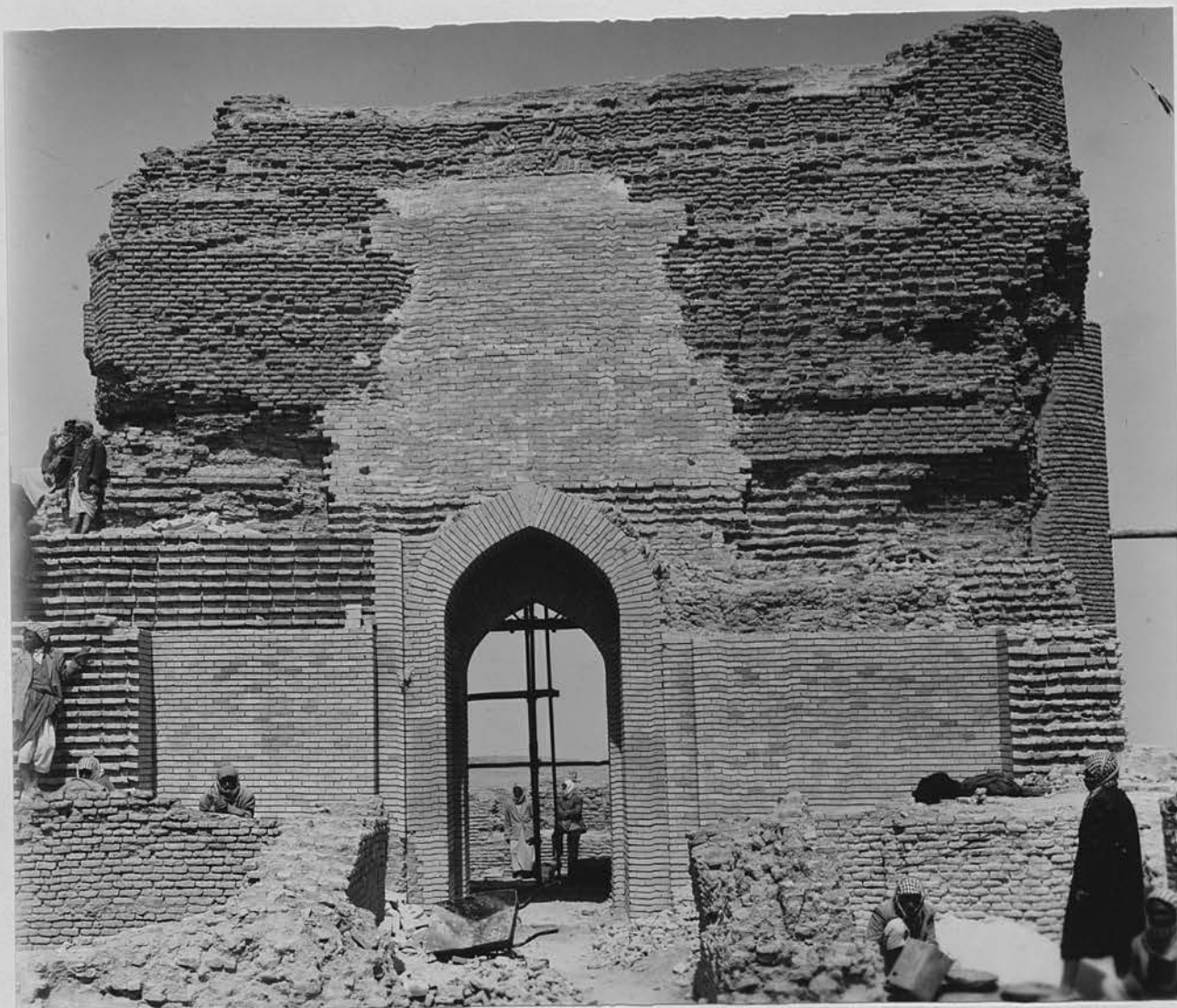
47. Wāsiṭ. Al-Madrassa al-Sharābiya (?): interior façade of the entrance during the course of restoration.
