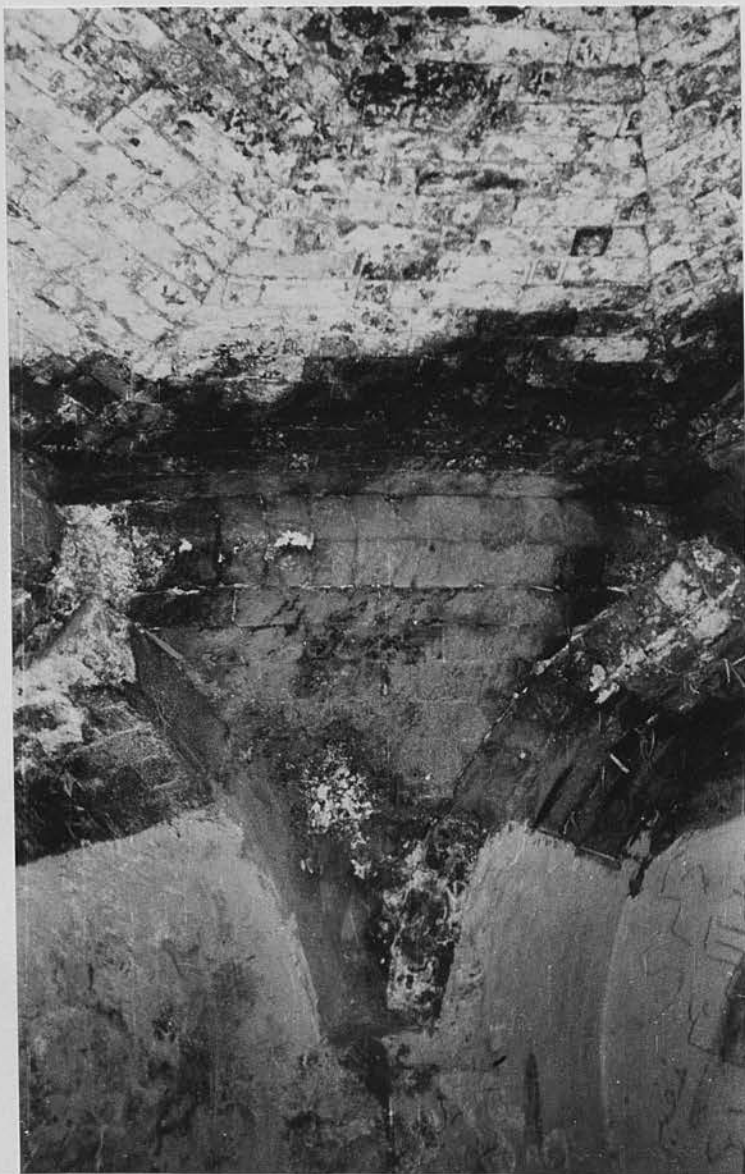
149b. Kūfa. Al-Sifīna: interior. Zone of transition of the south domical vault.
