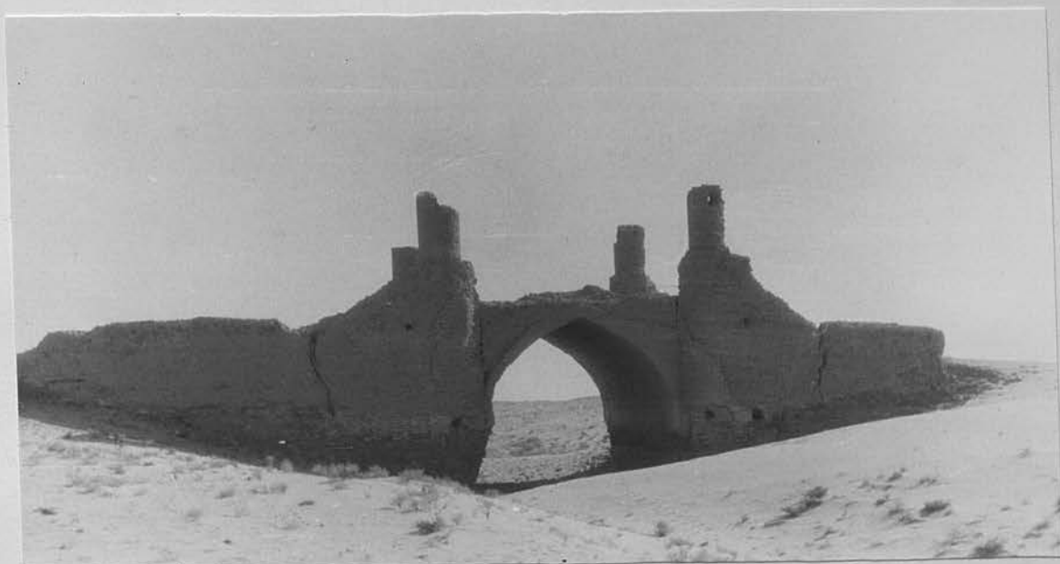
154b. Kūfa. The bridge of Kirī Si'da: north side.
