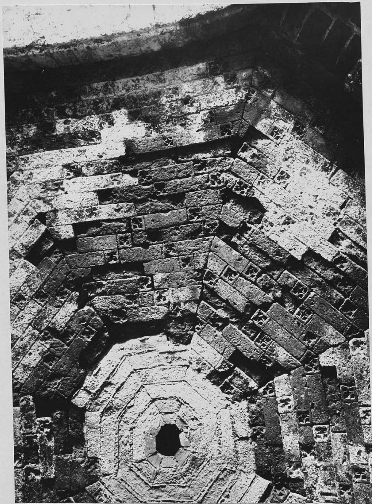
150. Kūfa. Al-Sifīna: interior. Detail of brickwork of southern vault.
