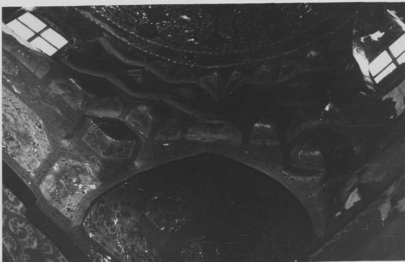
82a. Al-Kifl. The mausoleum of Dhū 'l-Kifl: interior showing zone of transition on north-east side.
