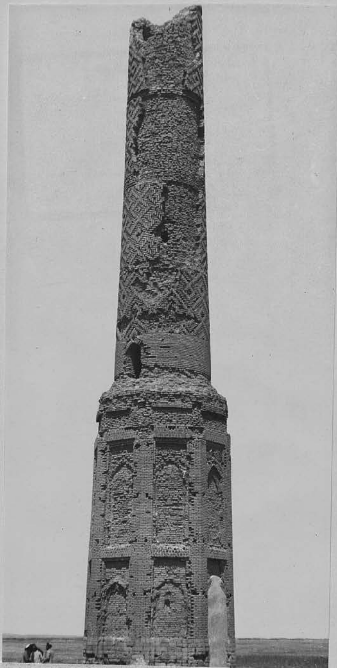
21. Arbīl. The minaret al-Muzaffariya before restoration.
