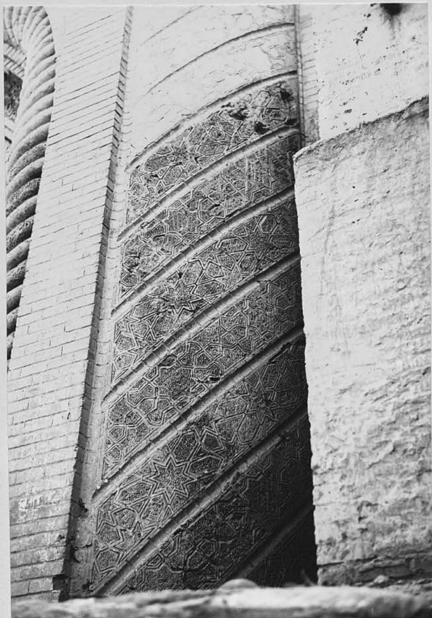
99. Baghdad. Al-Madrassa al-Mirjāniya: exterior. Main entrance: detail of the brick ornament on the right-hand side pier.
