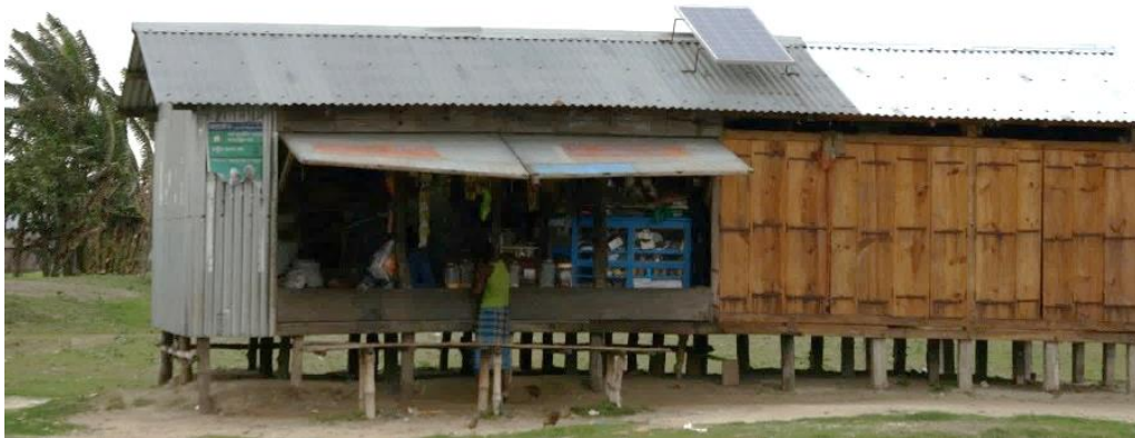
Picture 9: Newly installed Solar Panel on a Shop Roof
