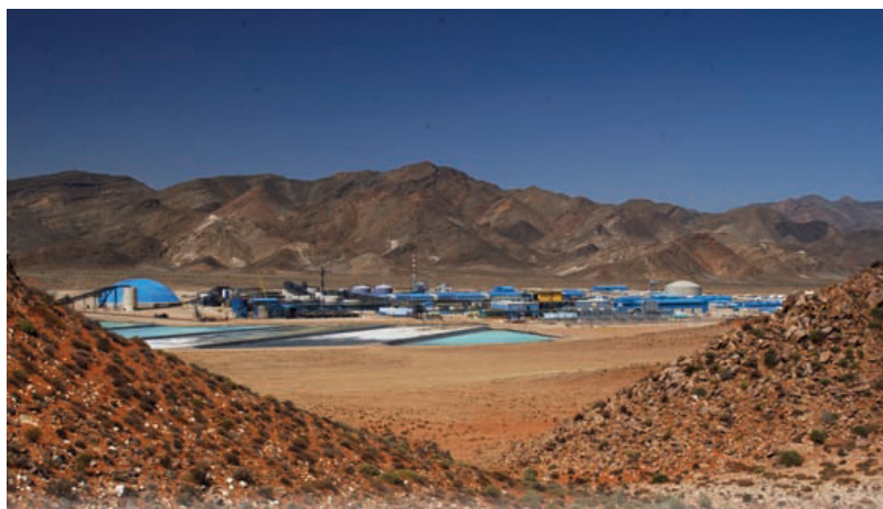
Figure 2.3: The Anglo American Skorpion Zinc installation in Namibia. 11
