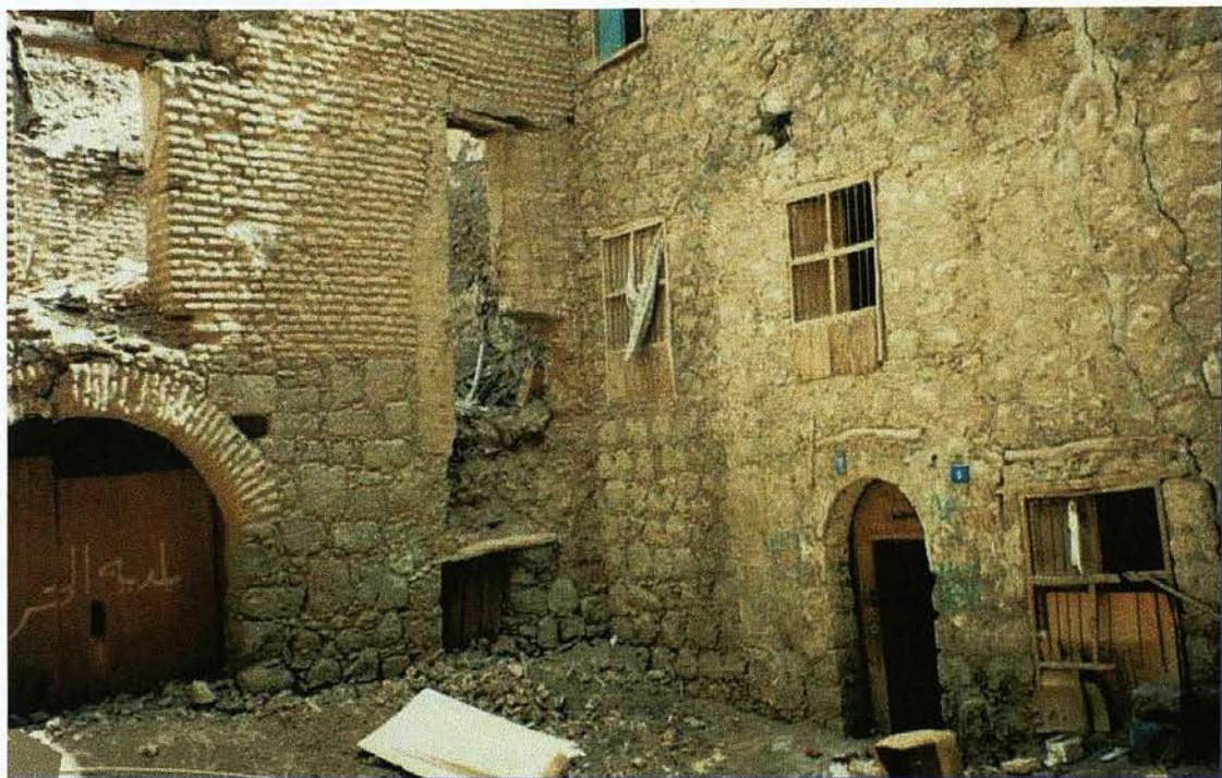
(08) A traditional two-floor building. This was built of mud with a roof made of parts of palm trees. This model is similar, to a great extent, to the old traditional buildings that spread in Madinah before Islam. This style continued to be used until very recently.
