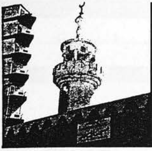
(52) The Northern side of the Abi Tharr Mosque.
