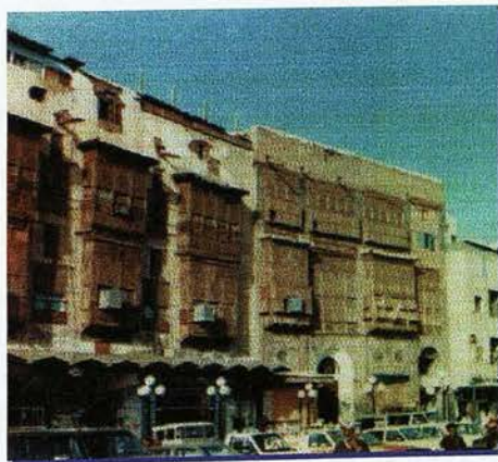
(01) Traditional houses in Madinah using local raw materials such as stone, mud and wood.
