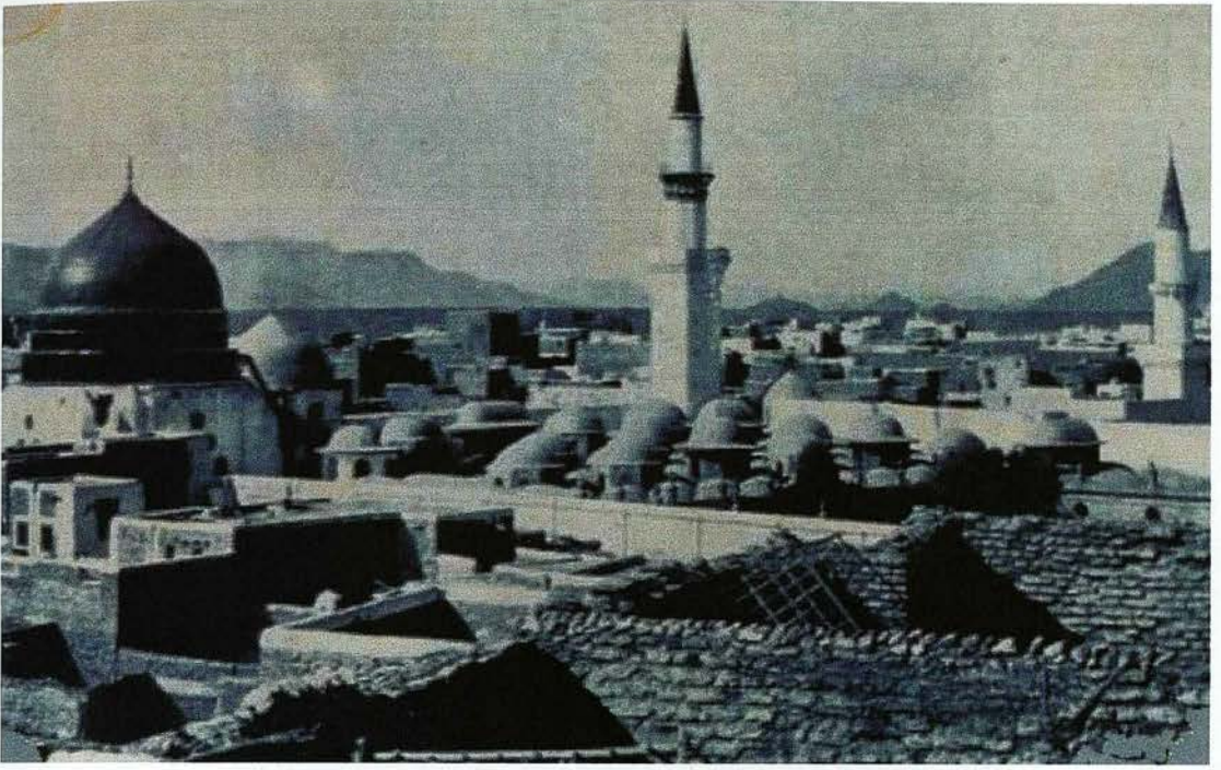
(22) The roof of the Prophet's Mosque, covered with a group of domes, the largest of which is the Honorable One, then the mihrab's. All of them are covered with lead. (53) ( Ministry of Information 1982 )
