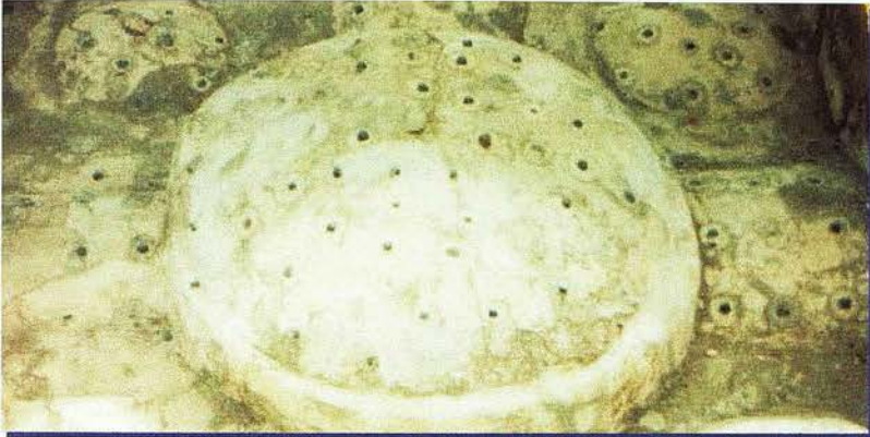
(44) Al-Anbaria bath (the roof).
